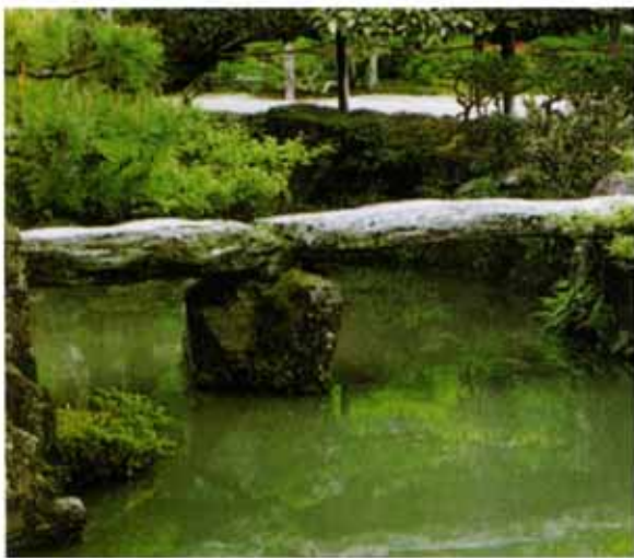
Senshu-hashi, the Bridge of the Hermit's Sleeve composed of two stone slabs in Ginkaku-ji Temple. Photo: Ken Kawai
