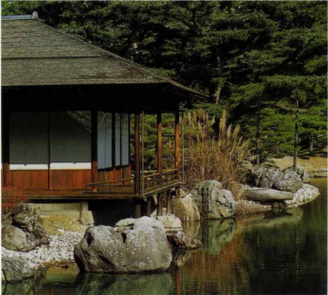
Rock foundations for the stilts supporting Kikugetsu-tei Pavilion in Ritsurin Park, Takamatsu.
