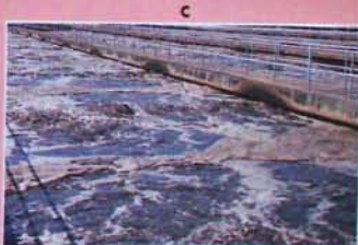
Microorganisms are used to degrade wastes and pollutants to maintain and restore environmental quality. An activated sludge treatment facility has tanks in which microorganisms degrade wastes. Extensive aeration and agitation maintain aerobic conditions that favor complete degradation of organic compounds by microorganisms.
