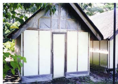
Figure 18. EPS (Expanded Polystyrene) growing house with polyethylene insulation and a bottom barrier along the ground (Photo courtesy of Tricita H. Quimio)
