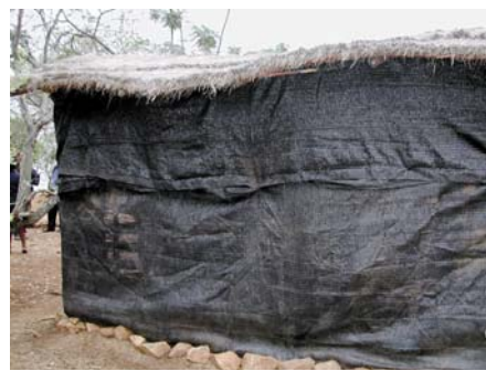
Figure 4. Thatch mushroom growing house draped by shade cloth and surrounded by a stone fence
