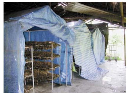
Figure 7. Steel structural tubing covered with tarpaulin
