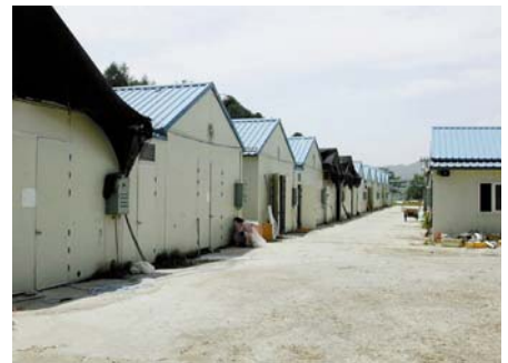
Figure 5. SIP (Structural Insulated Panel) house
