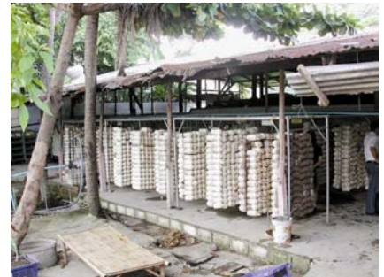
Figure 6. Steel frame structure with a roof
