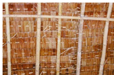
Figure 9. Bamboo pole rafter and
