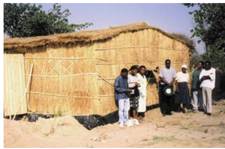
Figure 12. Rodent/snake barrier in the bottom part (Photo courtesy of Audrey R.S Mabveni)
