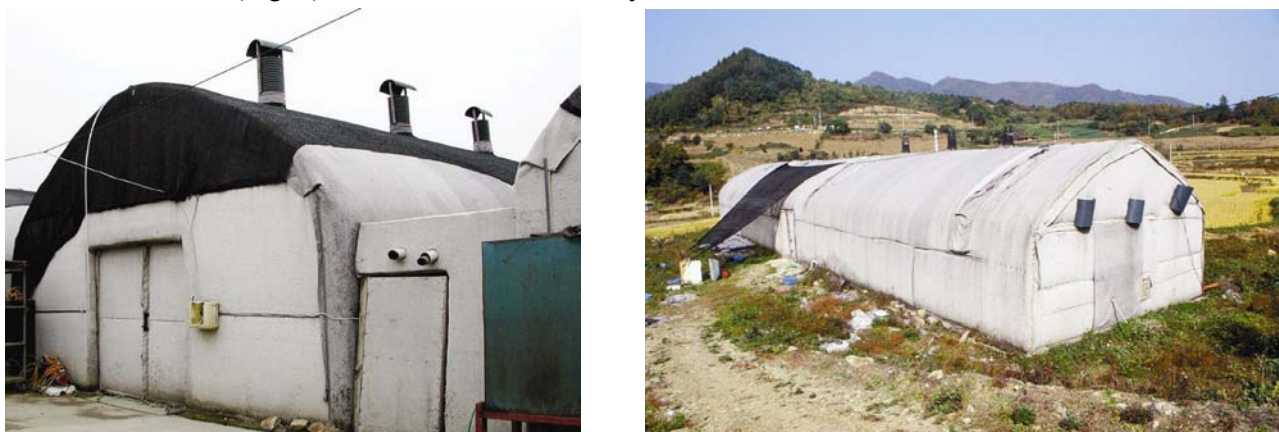
Figure 16, 17. Green house clad with insulation (glass wool) and roof vents
