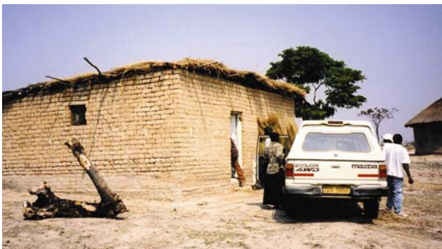
Figure 14. Brick house with a thatch roof and a vent house (Photo courtesy of Audrey)
