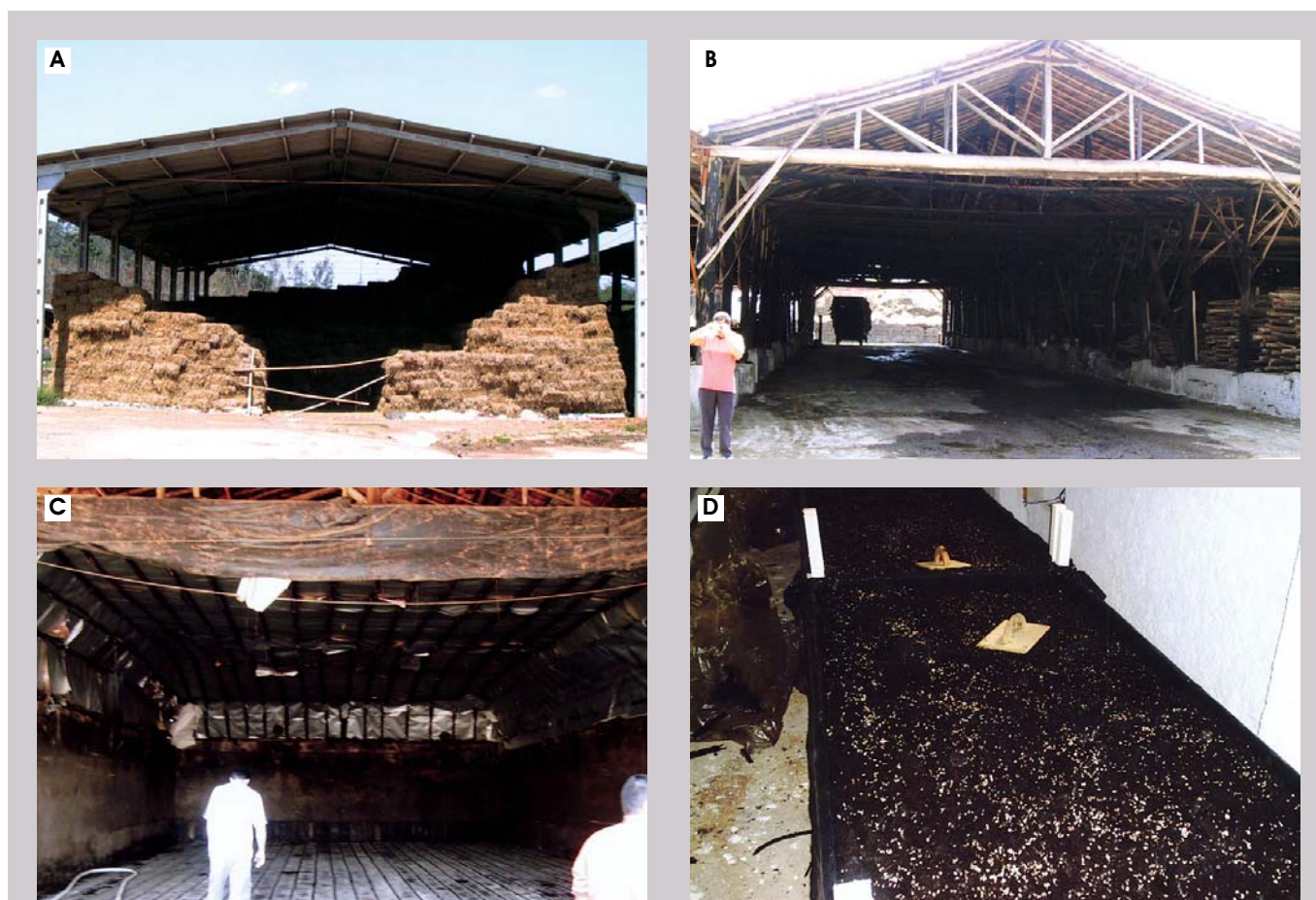
Figure 5. Composting unit in State of São Paulo A: Storage area of composting materials B: Fermentation area (phase I) C: Pasteurization room D: Compost inoculated at farmers growing house
