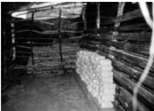
Figure 25. Bags laid on their side in row on the wall.
