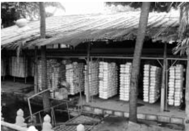
Figure 23. Simple structure for mushroom growing
