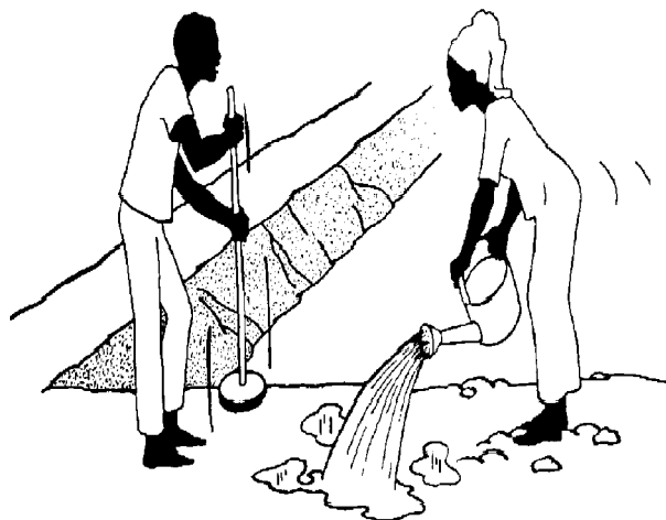
Figure 13: Compacting the dike (Viveen et al., 1985)
