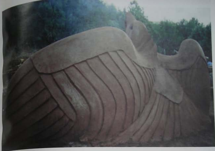
PHOENIX OVEN, REAR VIEW The site is an old lodge, recently revived as a B&B and educational center for natural building; thus a Phoenix rebirthing itself from the ashes. The oven is in the bird's belly, and smoke vents out the open beak.
