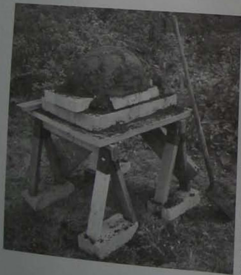
HELP! NO SAND: But plenty of topsoil, as this was in Minnesota, where the ancient floodplain of the Mississippi laid down topsoil tens of feet deep. A layer of newspaper would have helped when it was time to pull the form, but I didn't think of it. Since I also had no straw, I just decided to try making it out of pure clay subsoil, which I found in a nearby hillside. I fired it dry the next day, ready for baking!
