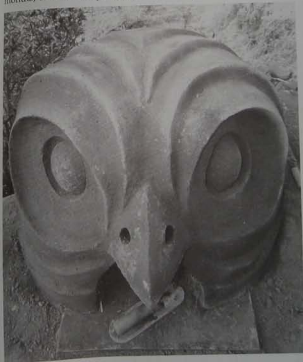
ATHENA'S OWL ARIZONA, 1996 A DESIGN THAT DIDN'T WORK The consequence of sacrificing practicality for aesthetics is frustration. The bird's beak was meant to vent smoke through the nostrils, but they are clearly too small, and provided no advantage in terms of extra draft. The mistake could have been ameliorated with a higher door, or different chimney design. (B. Steen Photo)
