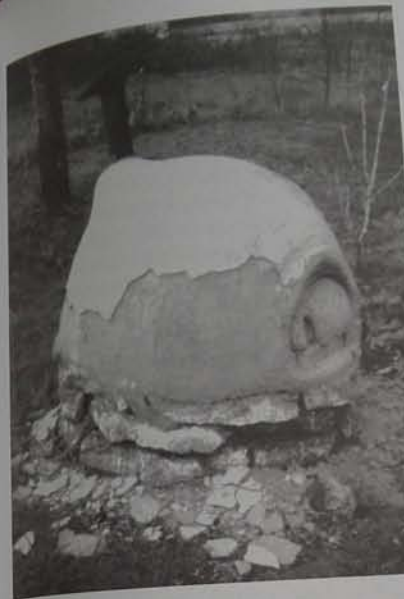
JASON'S OVEN AFTER A HARD WINTER note the beautifully molded door and handles, which were shaped out of lump of straw-ey cob and cement (for more on molded cob doors, see page 83).
