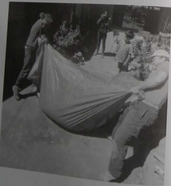
MIXING MUD WITH A TARP: Lean back, keep your spine straight — let your legs do the work. (B. Steen photo.)
