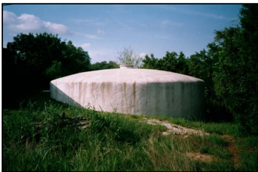
Figure 2-10. Ferrocement tanks, such as this one, are built in place using a metal armature and a sprayed-on cement.
