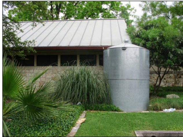
A 2,000-gallon, ranch-style metal cistern is one of two tanks that capture rainwater for landscaping at the Edwards Aquifer Authority building. (Photo courtesy: Lara Stuart)
