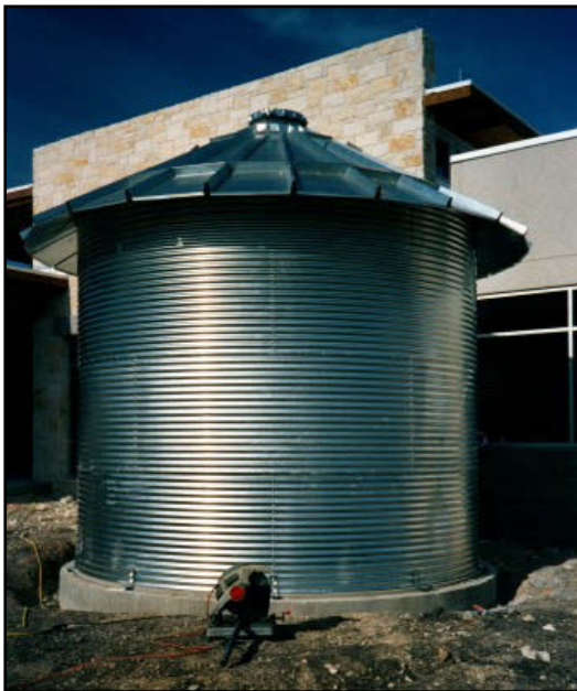
Figure 2-8. Galvanized sheet metal tanks are usually fitted with a food-grade plastic liner.
