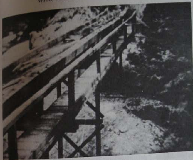
Logging Flumes in Neuburg
