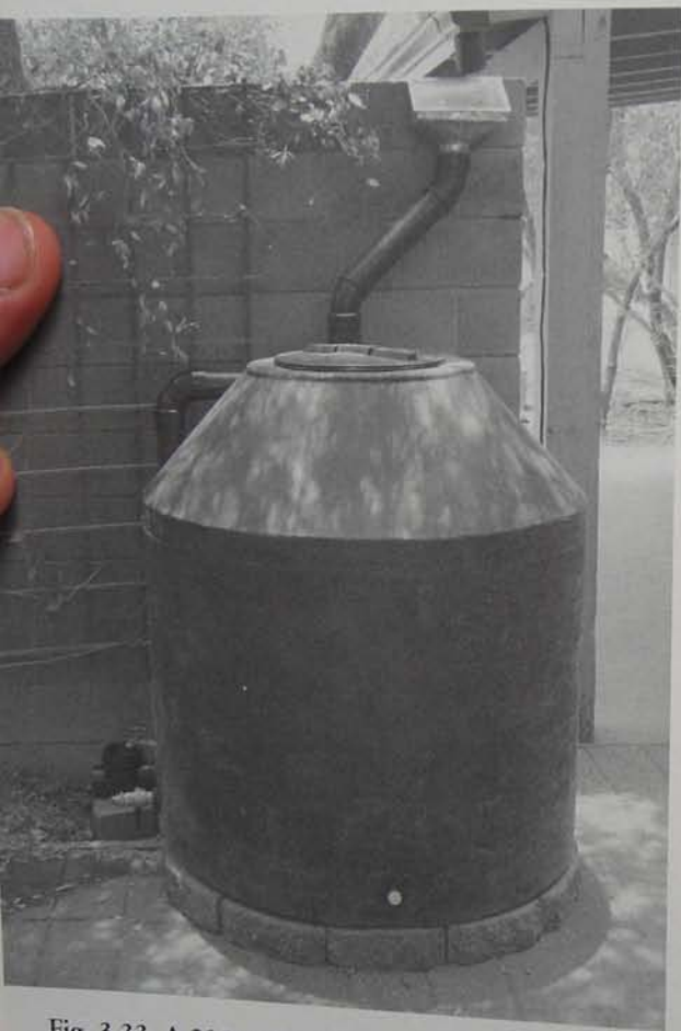
Fig. 3.33. A 305 gallon (1,159 liter) polyethylene tank with rainhead downspout screen collecting roof runoff from porch roof for courtyard landscape irrigation, Nature Conservancy offices, Tucson, Arizona. The two 45° bends in downspout pipe keep direct light out of tank. Access hole lid includes subtle vent. At bottom of tank on left side, a ball valve accesses tank water; beside the valve is a spigot accessing municipal water. Beside the spigot is the backwater valve directing overflow water to a mulched basin.
