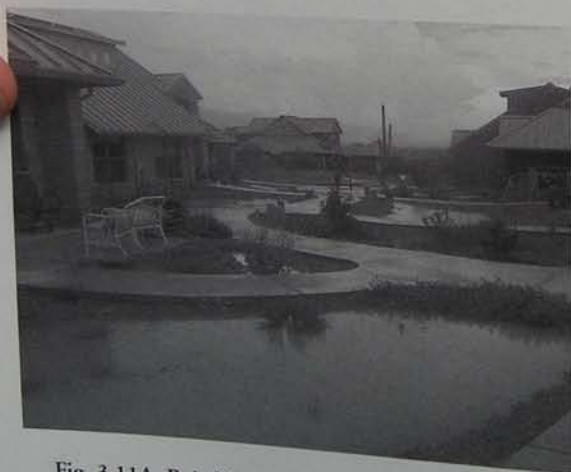
Fig. 3.11A. Rainfall collected in newly constructed infiltration basins minutes after a large summer storm. The basins have not yet been mulched or planted. Milagro Cohousing, Tucson, Arizona Credit: Natalie Hill
