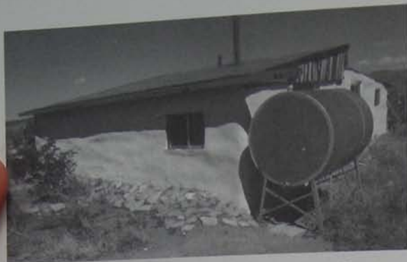
Fig. 3.36. The Howells' home and 500-gallon galvanized steel cistern
