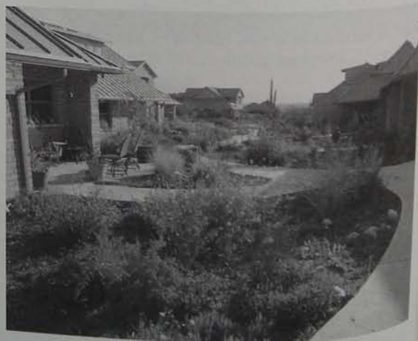
Fig. 3.11B. Same basins mulched and vegetated. Basins are designed to infiltrate water quickly so there are no problems with mosquitoes or anaerobic soils. These basins, with their spongy mulch and soil-burrowing plant roots, infiltrate all water within 20 minutes.
