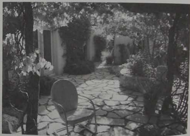
Fig. 3.18. A small yard with hardscape kept permeable by installing recycled sidewalk chunks with ample gaps for water infiltration, Amado residence, Tucson, Arizona
