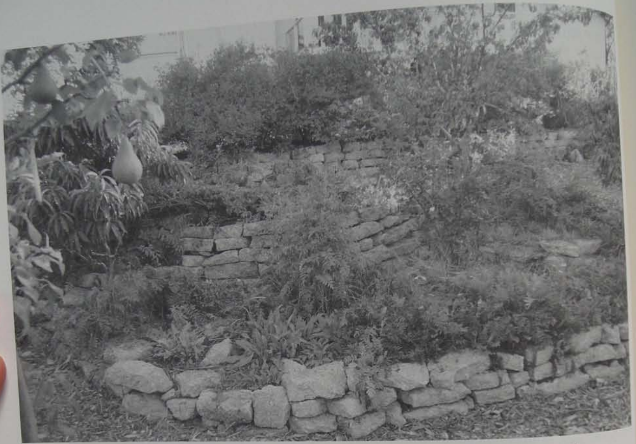
Fig. 3.5. Terraces stabilized with salvaged concrete retaining walls in the sloped backyard at the Zemach residence, Los Alamos, New Mexico
