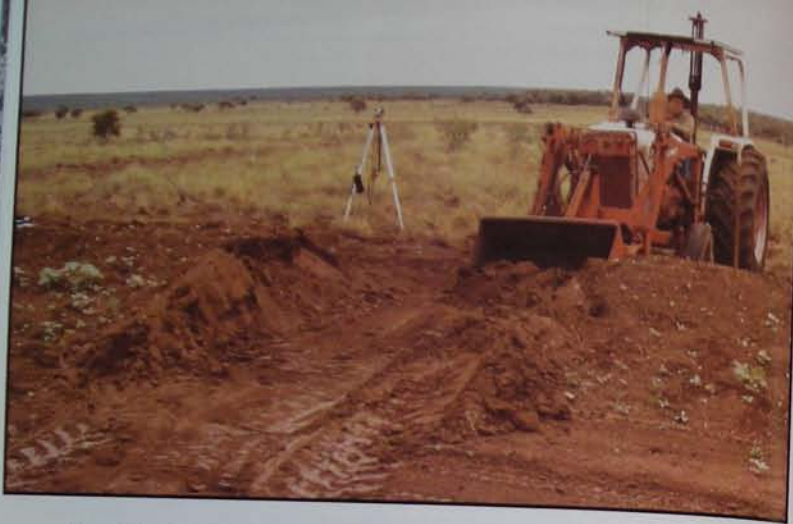
Plate 51 A front end loader is used to remove a section of a Flood-flo irrigation channel's bank for the installation of a water gate.
