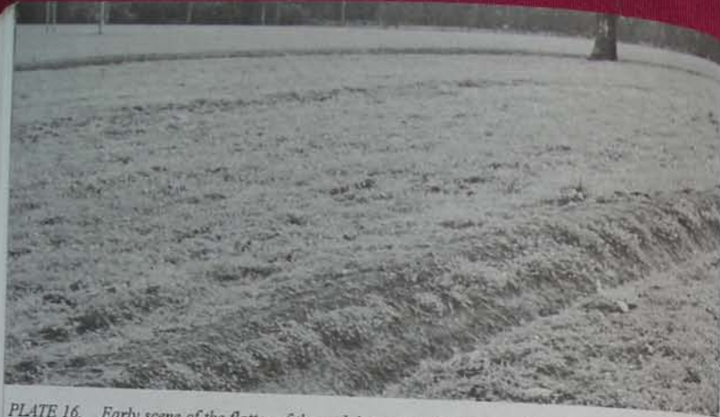
PLATE 16. Early scene of the flatter of the undulating land of "Yobarnie" showing an irrigation channel in the foreground. It carries 1.4 megalitres (300,000 gallons) of water per hour on a fall of 1 in 300; irrigation rate is 2.4 ha (six acres) per hour controlled by irrigation flags. Channel width at ground level is 1,120 mm (44 inches). This area was later subdivided into small paddocks. A fence parallels the irrigation channel. It is positioned at least 6.4 m (21 feet) above it. The up and down fences are on the lines of maximum fall. The lower line is part of the creek diversion channel.
