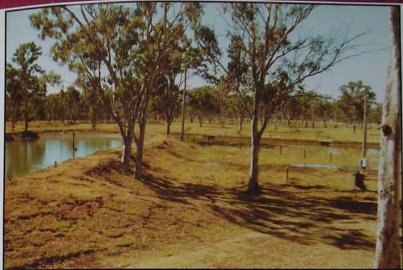
Plate 49 Panorama continuing from previous page. Flood-slo contour channel can be glimpsed wrapping around dam. When full, the channel inundates back to the wall. Steering banks can be seen beyond the channel.
