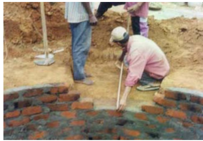
Figure 6: Measurement taken for the inlet construction
