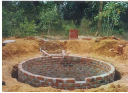
Figure 11: Completed tank before plastering
