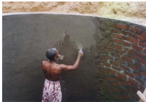
Figure 12: Plastering the tank
