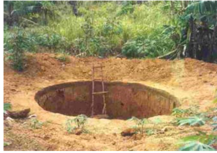
Figure 3: Pit for the tank construction
