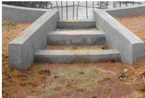
Figure 9: Inlet of the run off tank after plastering
