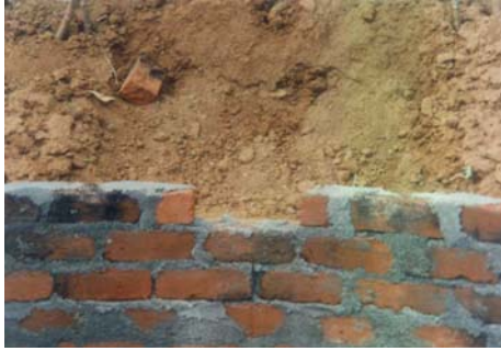
Figure 10: Outlet of the tank
