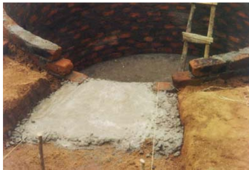
Figure 7: Concrete base for the inlet construction
