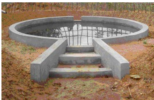
Figure 14: After the completion of the rainwater-harvesting tank
