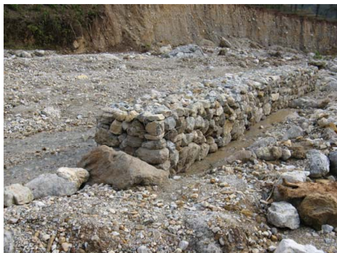
Figure 6: An example of a spur that has not been installed with groundwork or an apron and consequently is likely to be washed away during heavy flooding.
