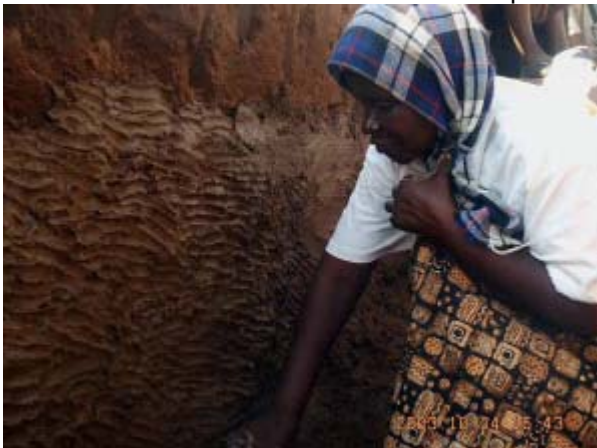
Picture 3: Tank lining/ Plastering ©Practical Action/Douglas Gumbo
