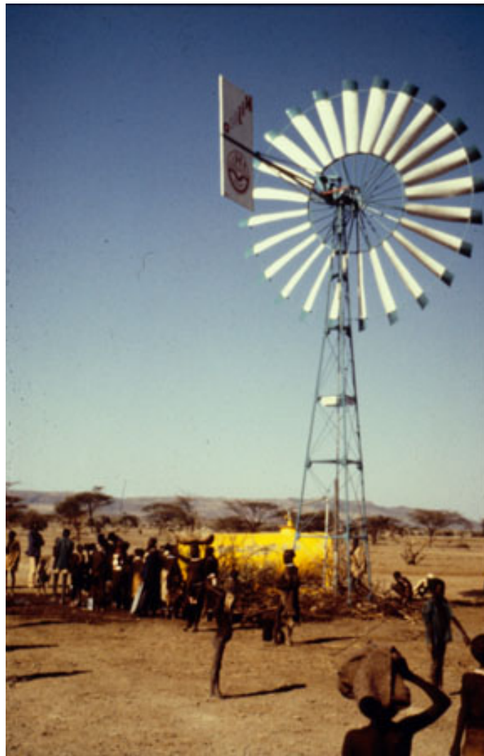
Figure 3: The Kitjito Windpump. Used to pump ground water in the Bhel region of Turkana for the Nomadic Pastoralists ©Practical Action
