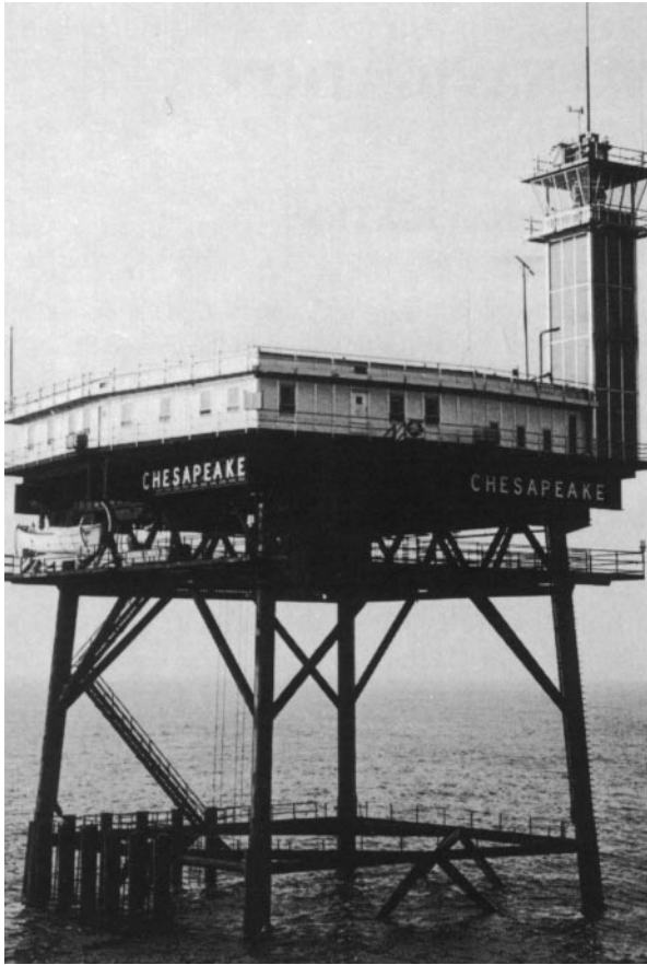
Figure 501a. Typical offshore light station.
