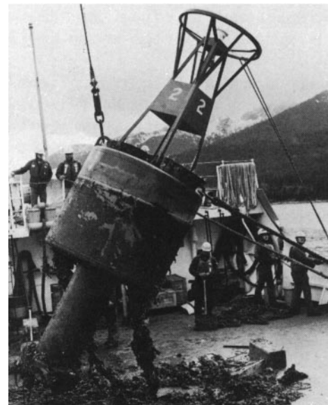
Figure 509. Buoy showing counterweight.
