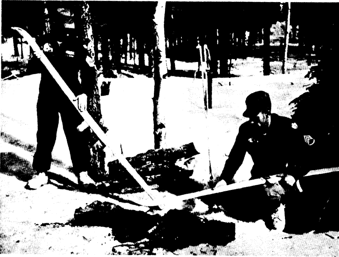
Figure 4-6. Heating skis over an open flame.
