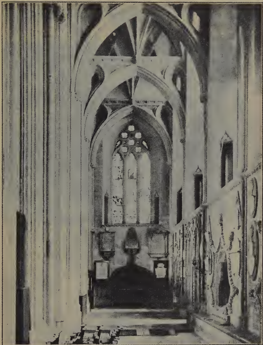
OPEN-WORK VAULTING AT BRISTOL.
