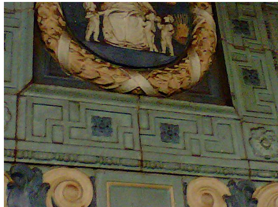
Figure 99: Subway station wall with svastika, NY.
