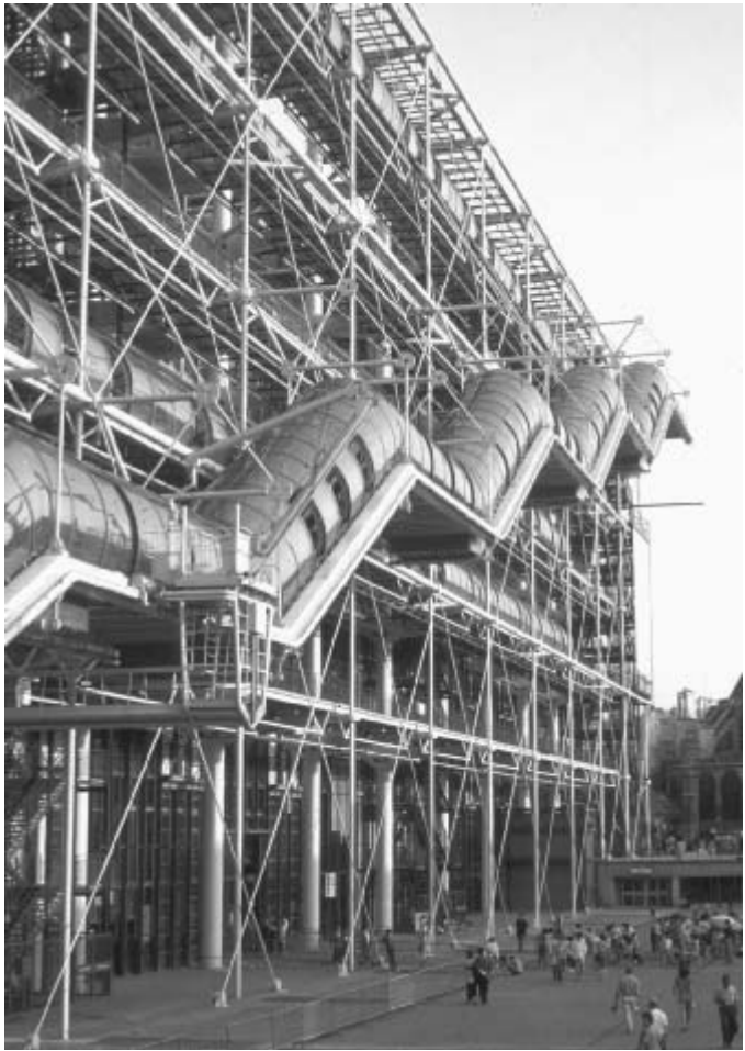
Figure 10-16 High tech structure: Pompidou Center, Paris, by Piano and Rogers (FH).
