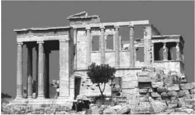
Figure 5-10 Use of the Ionic order for an irregular plan: Erechtheum, Athens (courtesy Ann Thomas Wilkins).
