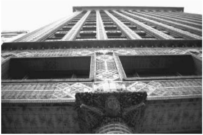
Figure 10-6 Space-cage frame: Guaranty Building, Buffalo, by Adler and Sullivan (courtesy Kai Gutschow).
