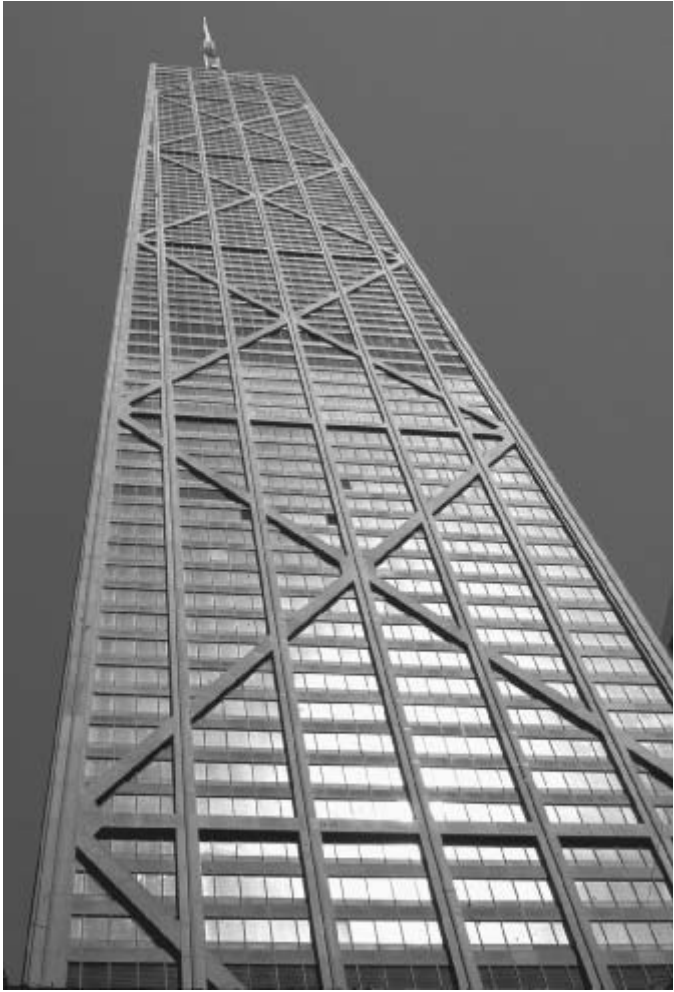
Figure 10-8 Diagonally braced external frame: John Hancock Center, Chicago, by Skidmore, Owings & Merrill (FH).
