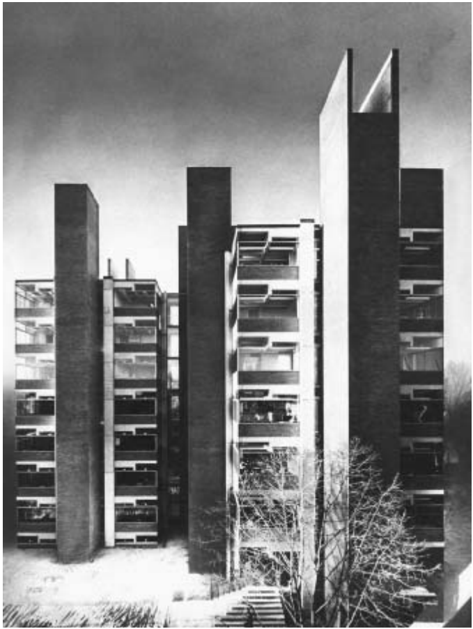
Figure 9-20 Distinction of “servant” and “served” spaces: Richards Biological Sciences Laboratory, University of Pennsylvania, Philadelphia, by Kahn (Malcolm Smith, for the Louis I. Kahn Collection, University of Pennsylvania and Pennsylvania Historical and Museum Collection).
