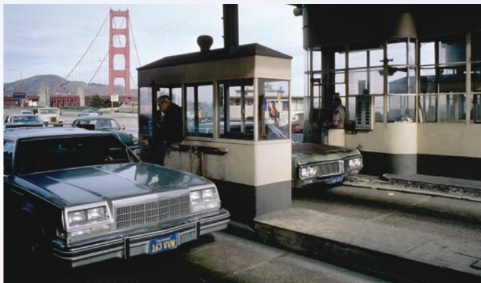
Toll plaza at the Golden Gate Bridge, San Francisco
