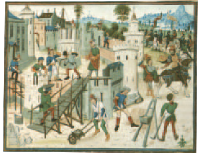
MEN AT WORK Workers supply stone blocks using a wooden ramp and a type of wheelbarrow. Often rough stone-and-mortar walls were faced with ashlar. If the whole wall was not faced, ashlar would be put around doors, windows, and loopholes.
