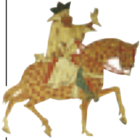
CONQUERING KING Edward I was a great builder of castles in north Wales.
