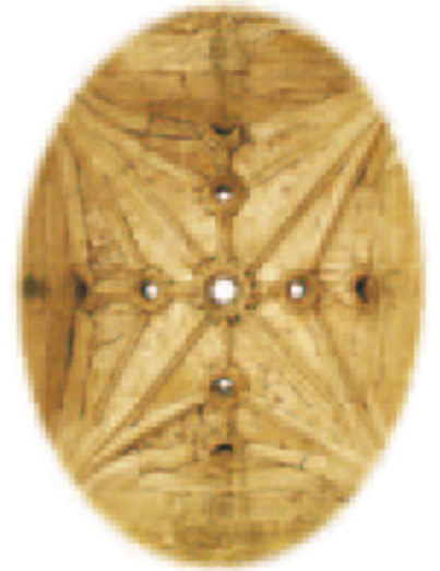
DROPPING IN The gate passage at Bodiam has so-called "murder holes" ( neutrières ) in the roof so cold water could be poured down to put out fires. Scalding water, hot sand, or other offensive substances might be also dropped on enemies who managed to get in.
