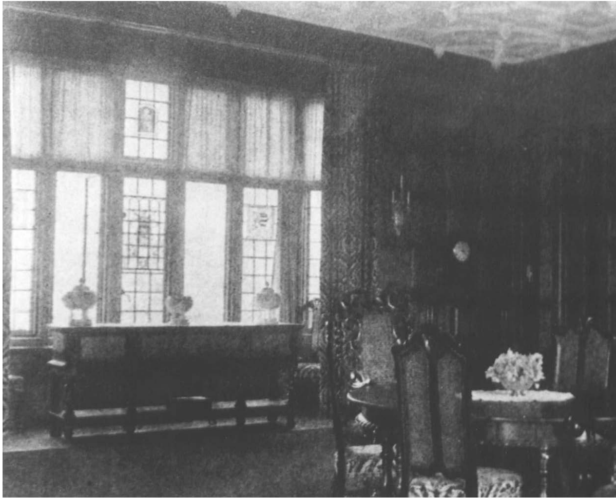
7. The dining room at George D. Pratt's estate, Killenworth, at the beginning of its occupancy (from Country Life 1914, p. 39)
