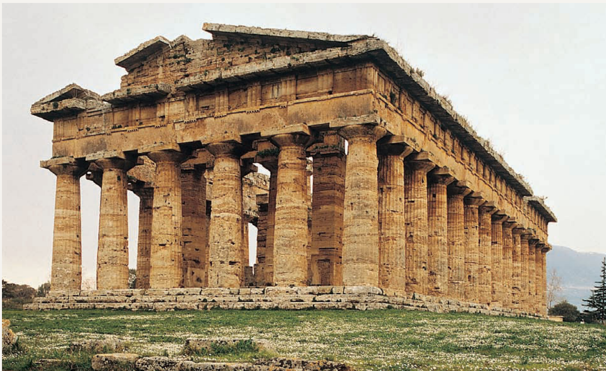
Greek Doric peripteral temple (Temple of Hera II, Paestum, Italy, ca. 460 BCE)
