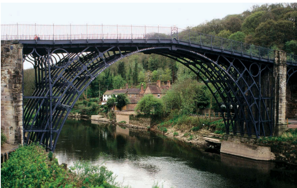
21-11 ABRAHAM DARBY III and THOMAS F. PRITCHARD, iron bridge, Coalbrookdale, England, 1776–1779.
