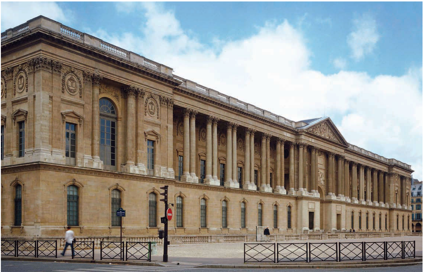
20-31 CLAUDE PERRAULT, LOUIS LE VAU, and CHARLES LE BRUN, east facade of the Louvre, Paris, France, 1667–1670.
