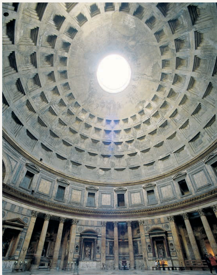
Roman dome with oculus (Pantheon, Rome, Italy, 118–125)
