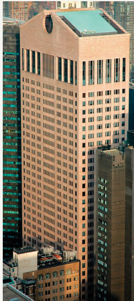
25-64 PHILIP JOHNSON and JOHN BURGEE (with SIMMONS ARCHITECTS), AT&T (now Sony) Building, New York, 1978–1984.
