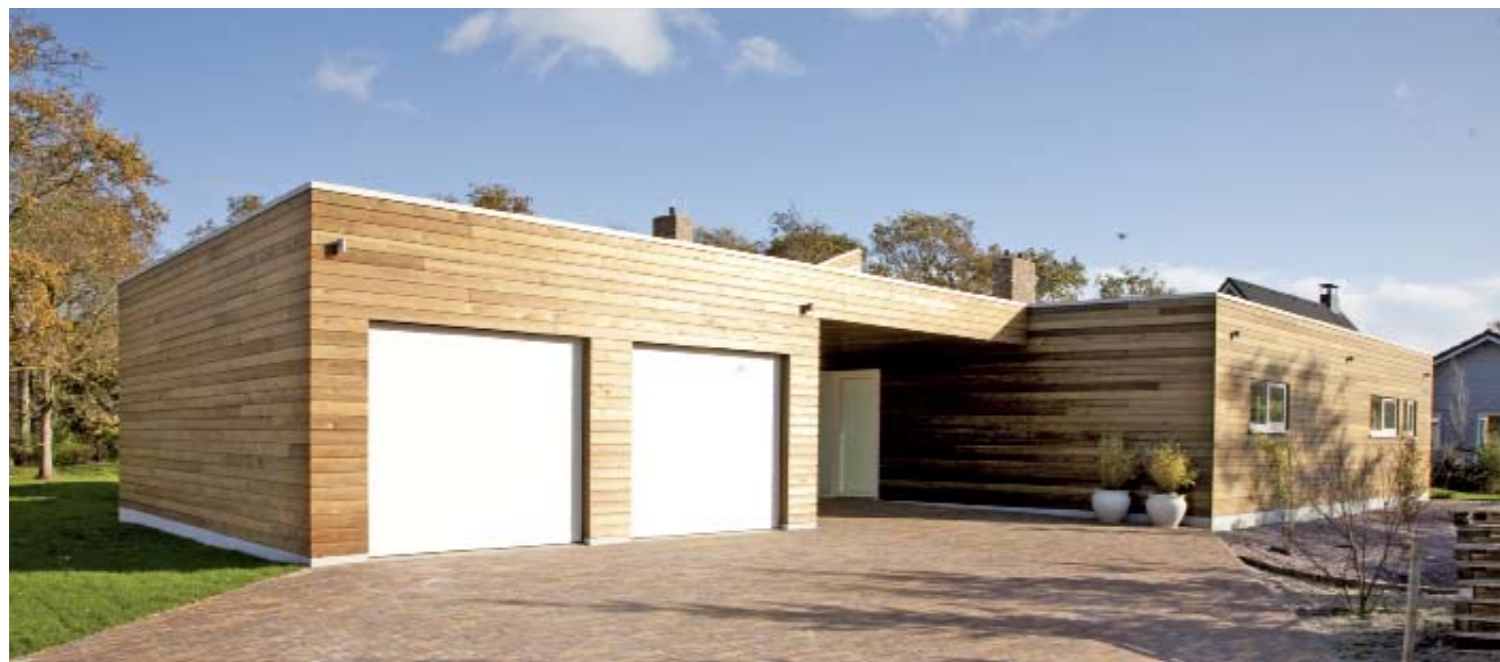
Entrance façade, Southwest
