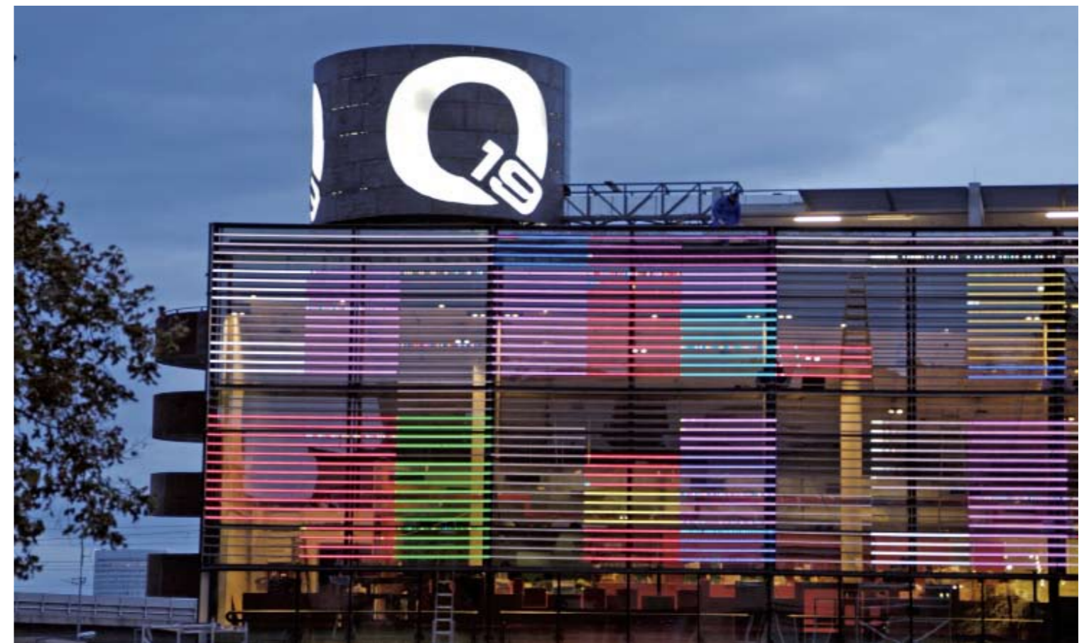
Façade – LED façade, entrance
