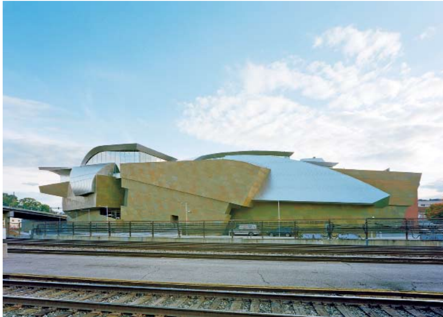
Exterior View of North Façade
