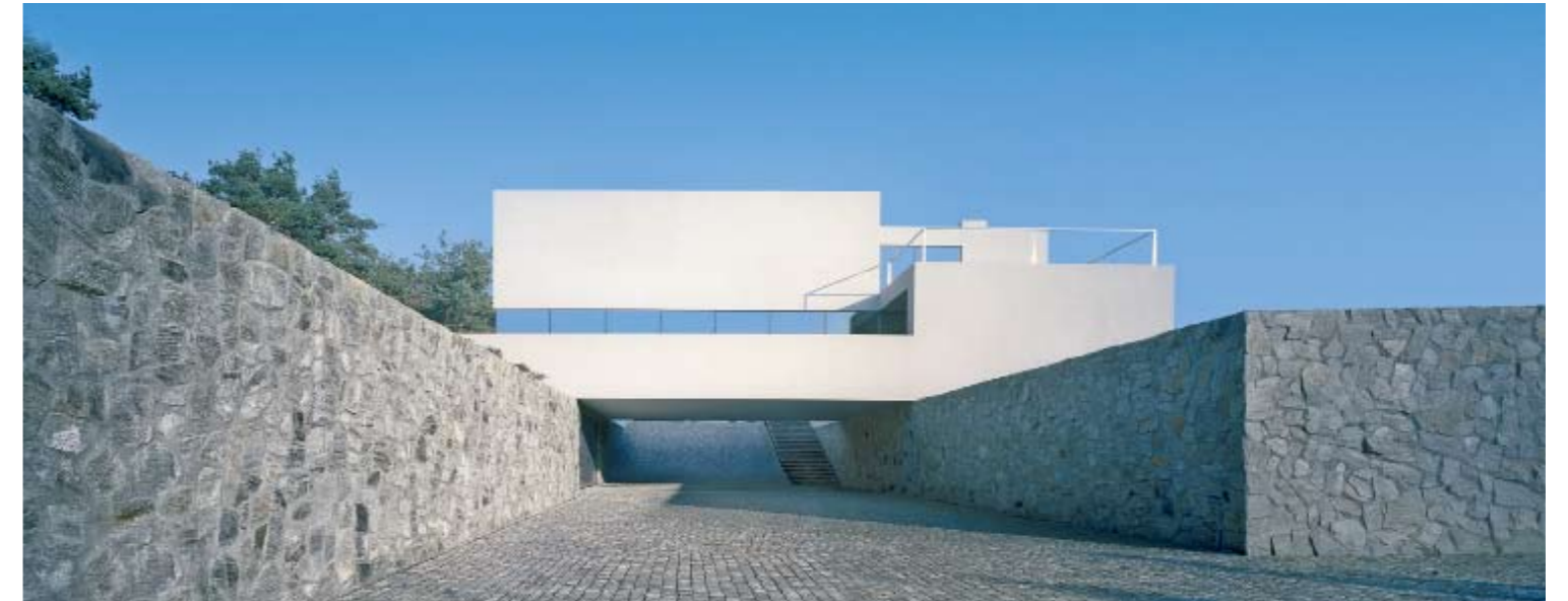
A view of the driveway leading inside to the ground floor level
