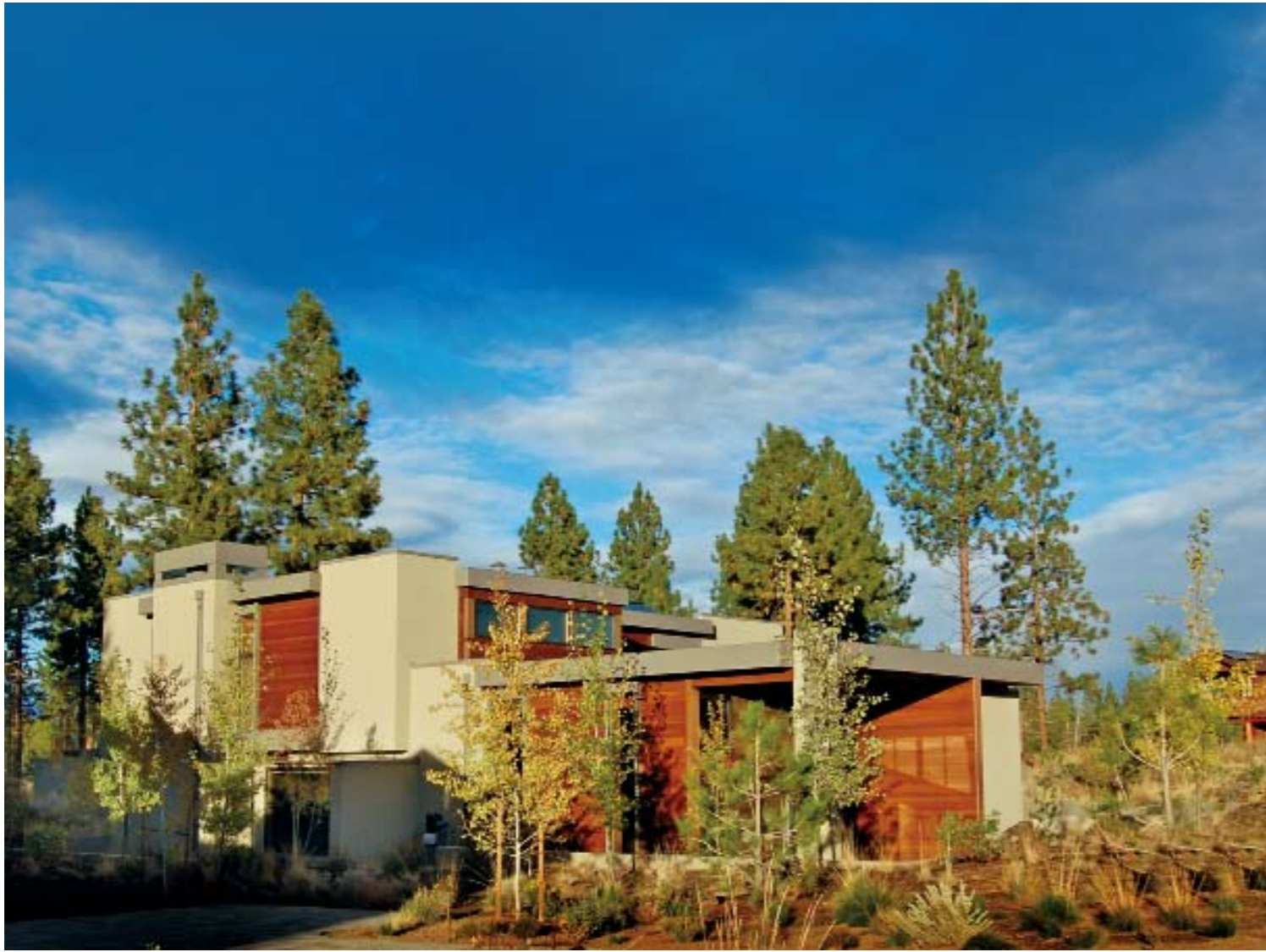
Building in the evening
