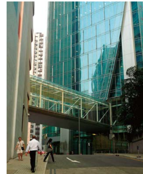
Footbridge to OIE
