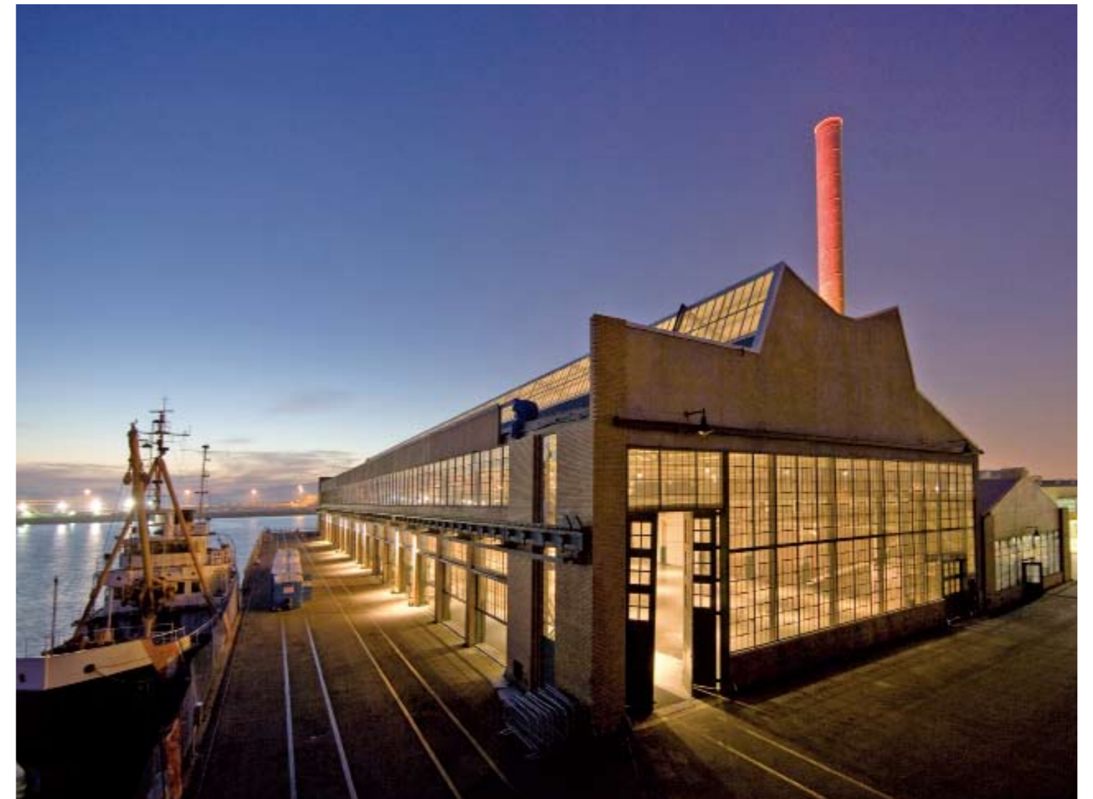
Craneway and Boilerhouse exterior
