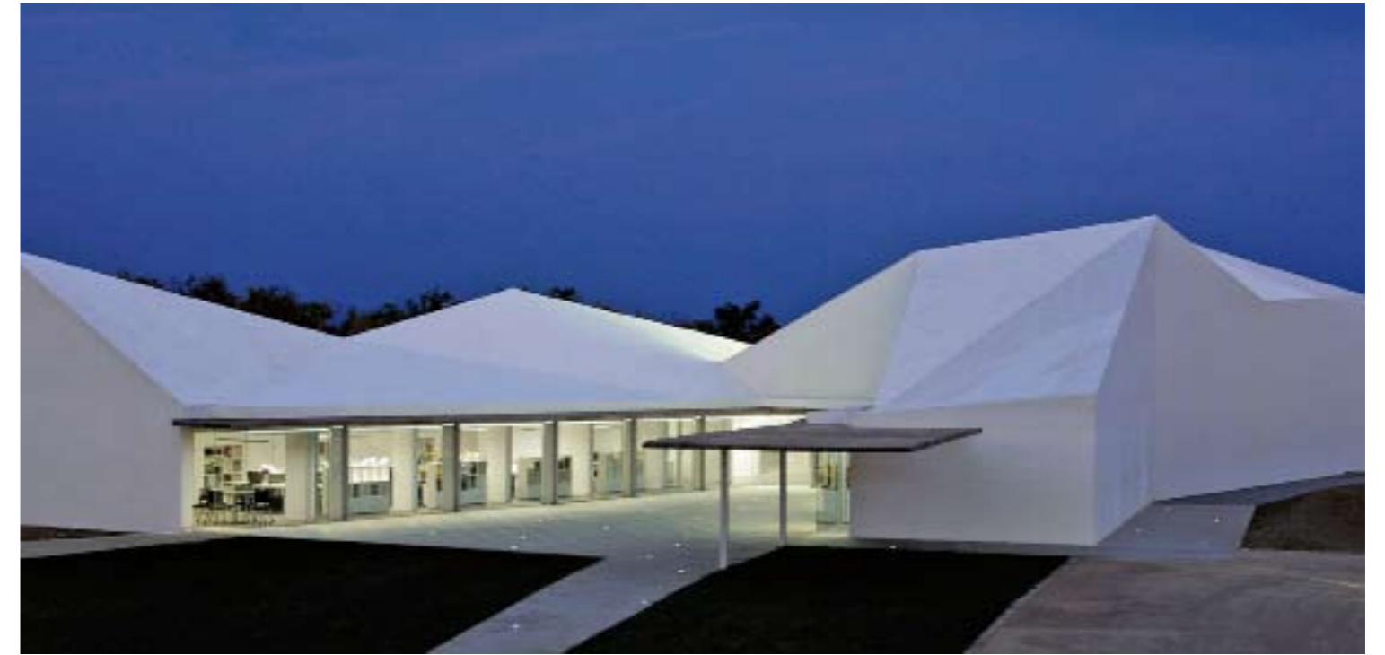
Night view of the exterior
