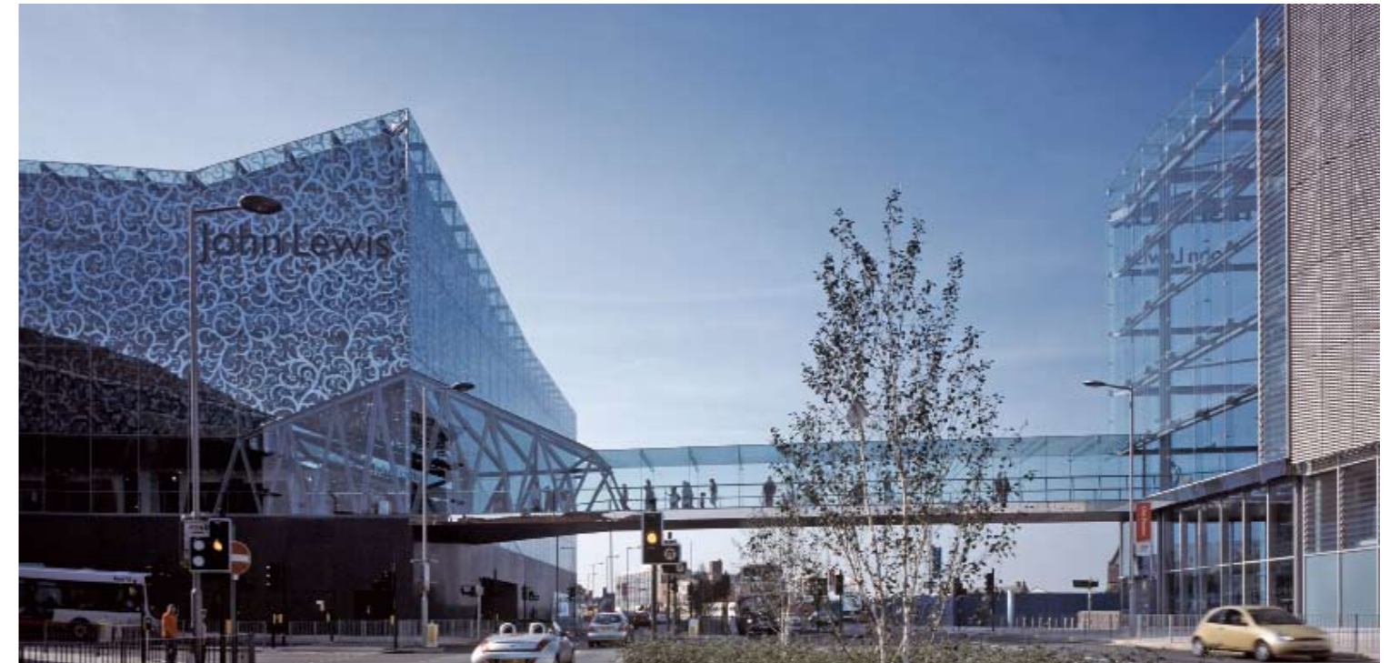
Façade with bridge
