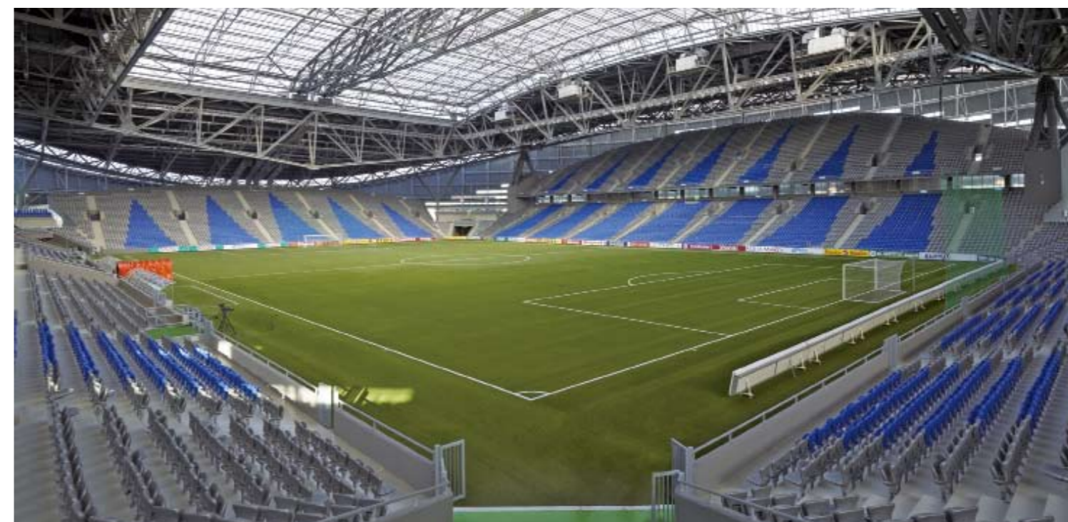
Operable roof system over the elliptical outer form
