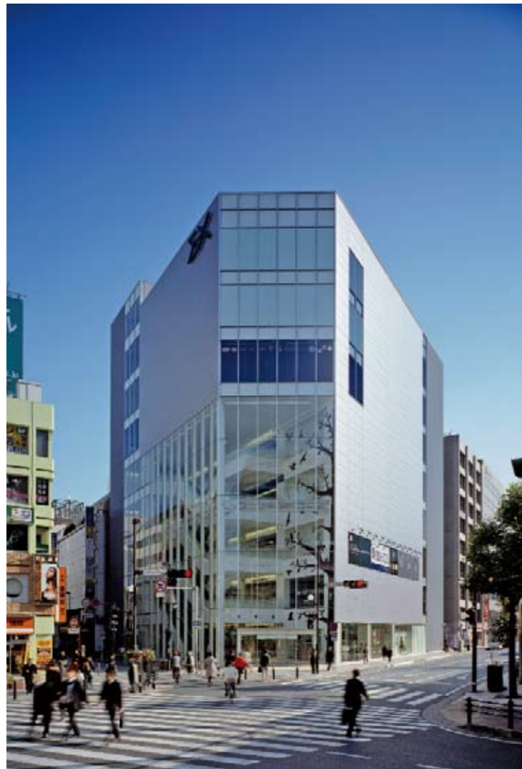
Looking towards the elevation facing the scramble junction
