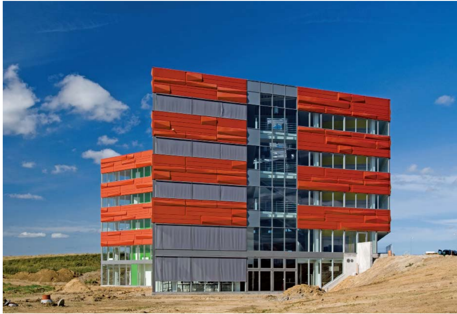
View from the south
