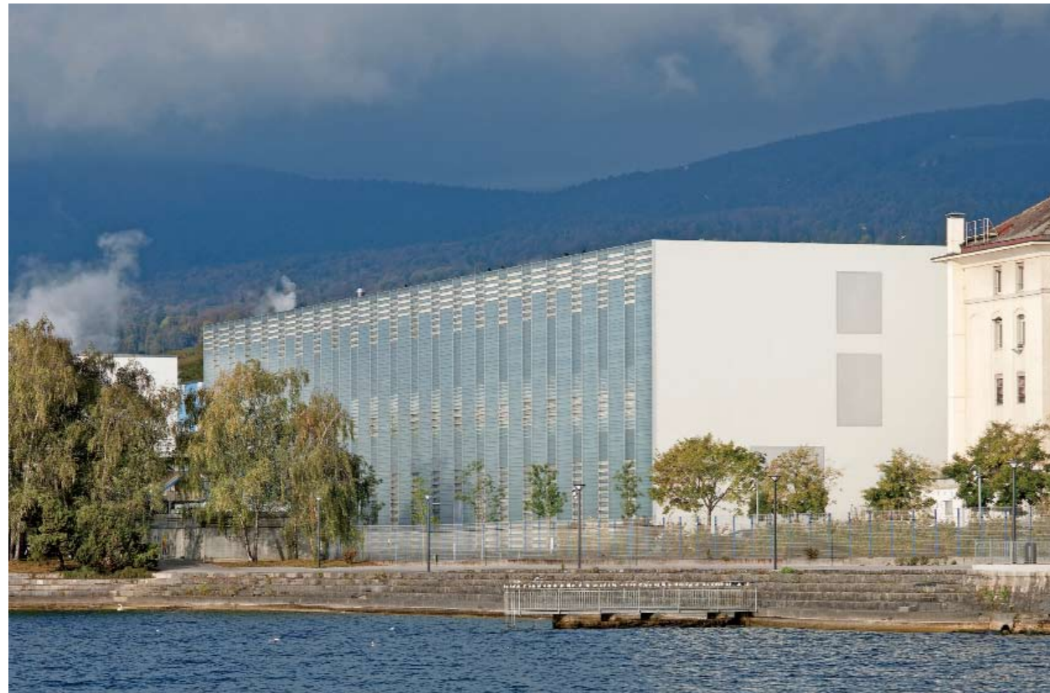
South Façade, took from the Neuchâtel Lake
