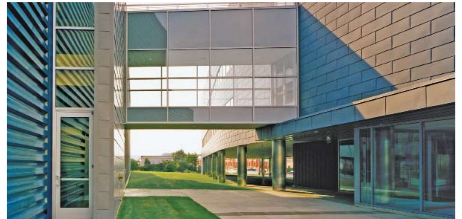
View of connecting corridor between office and manufacturing building
