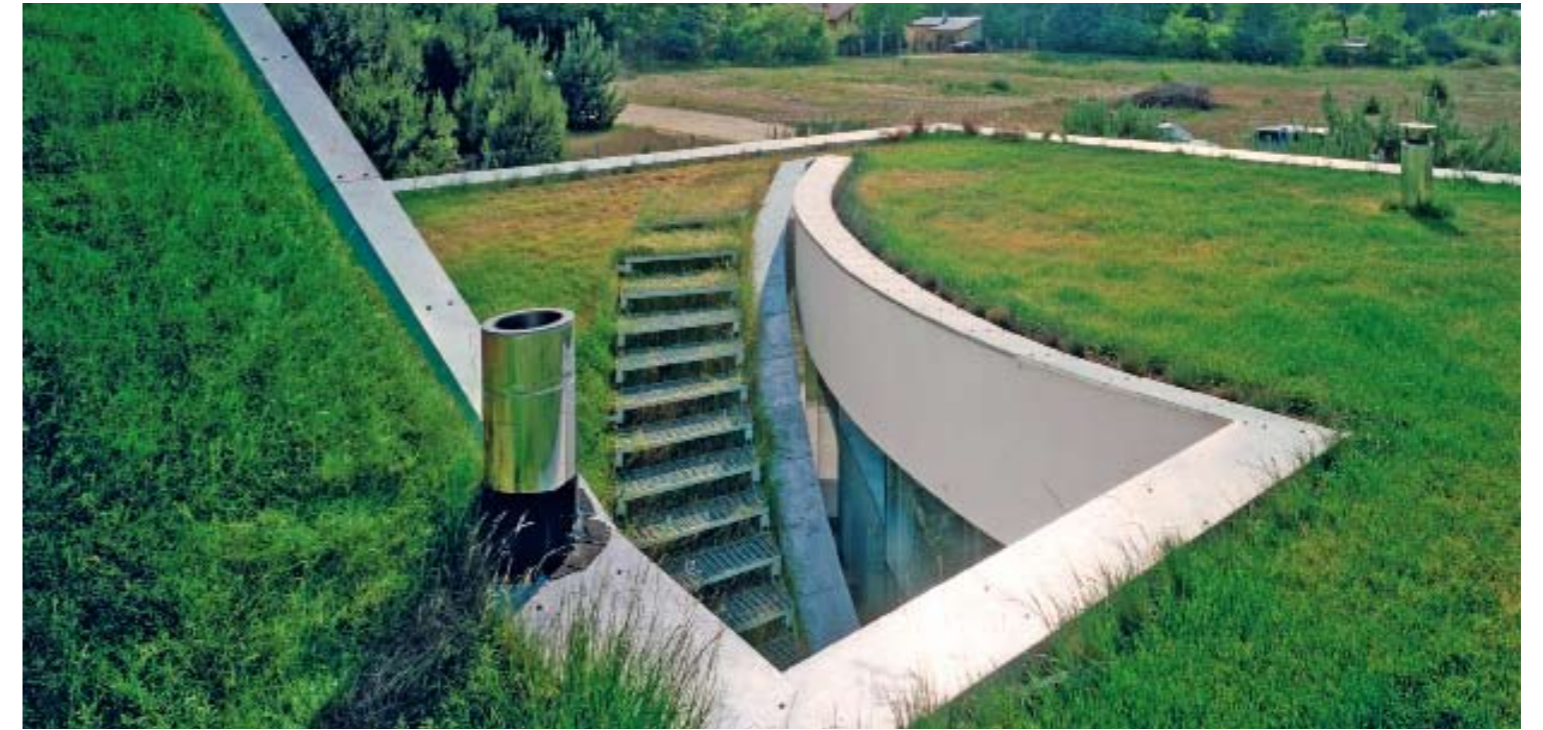
The stairs leading to the roof with one mesh across which grows the grass
