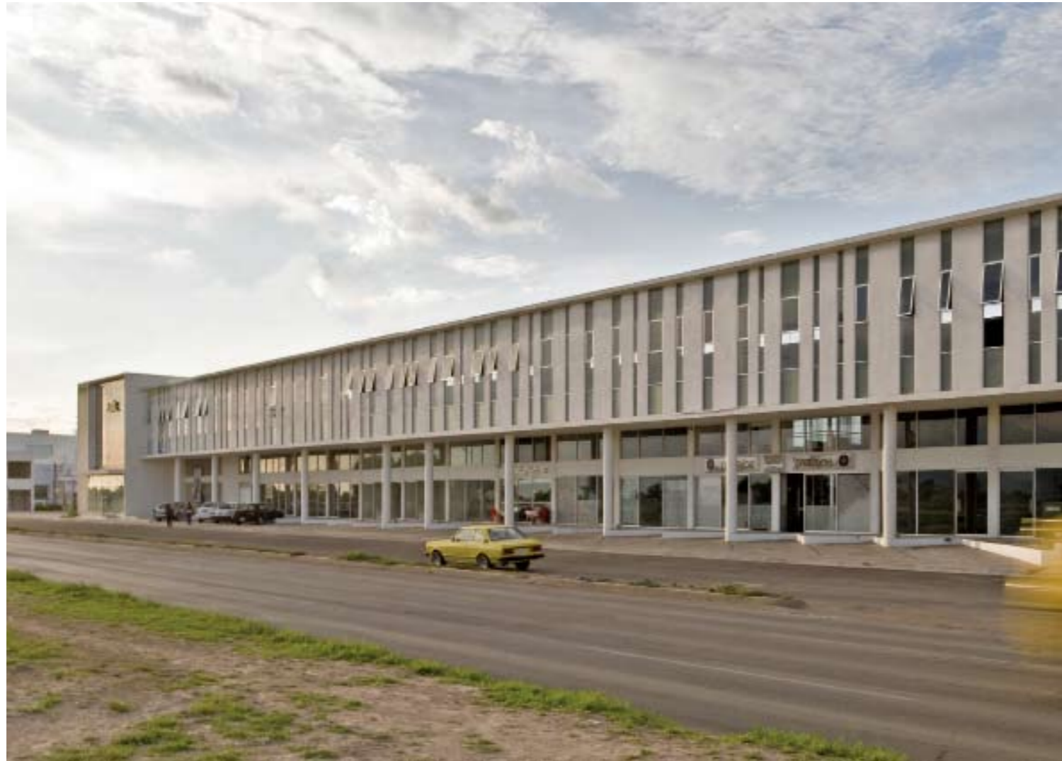
It is an almost 100-meter-long building, with a series of vertical strips used for ventilation by tip-up windows
