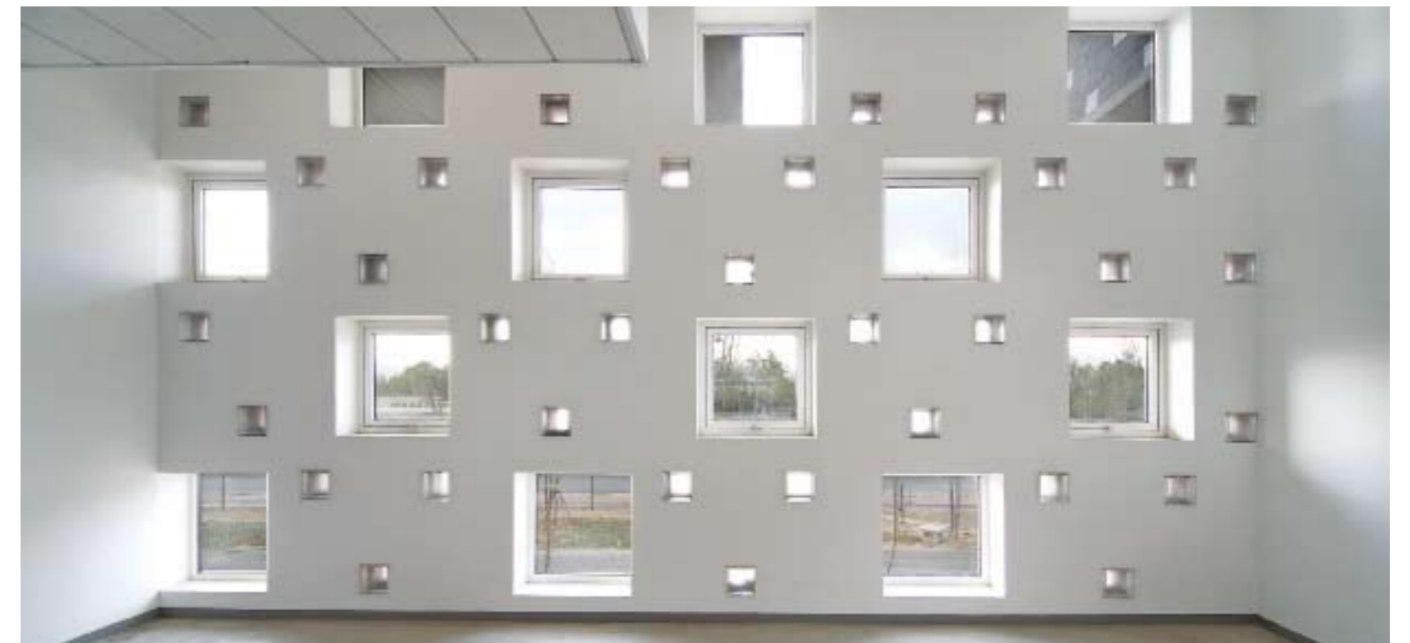
Inside of wall
