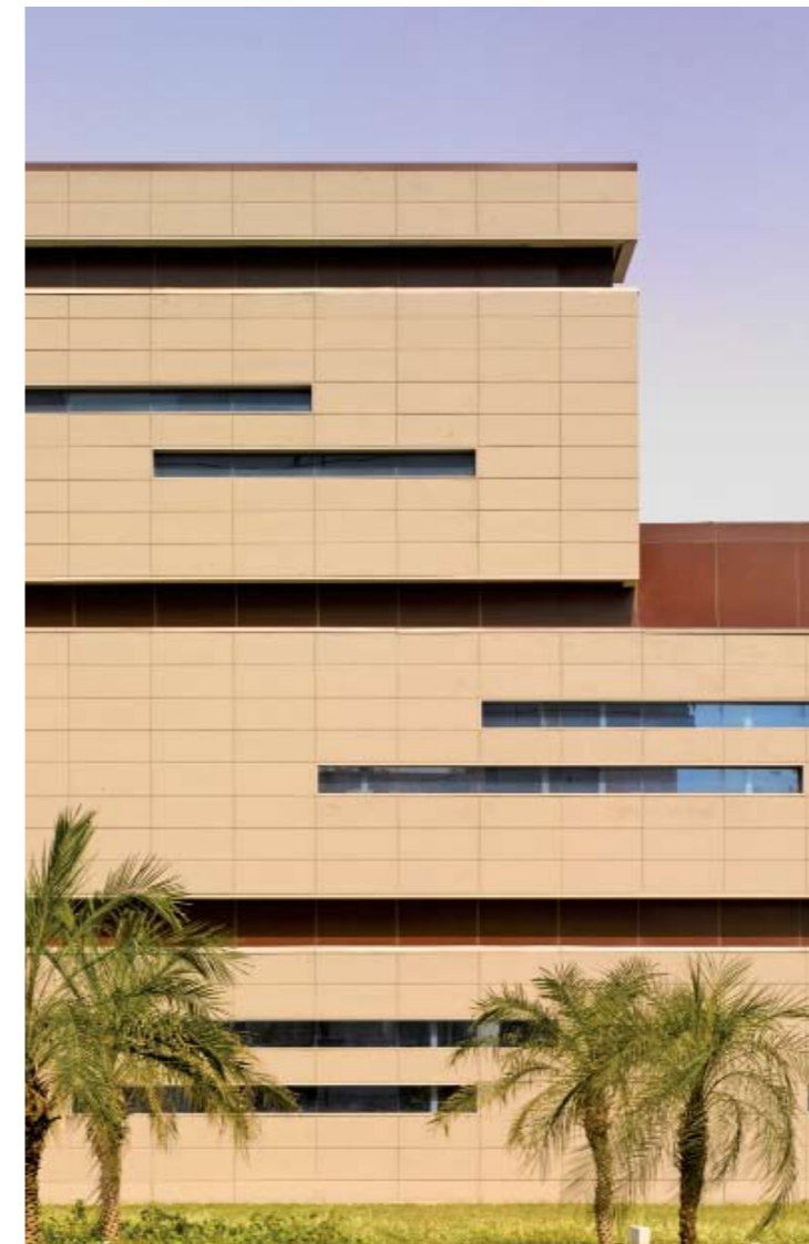
Shaded outer façade with small slit windows
