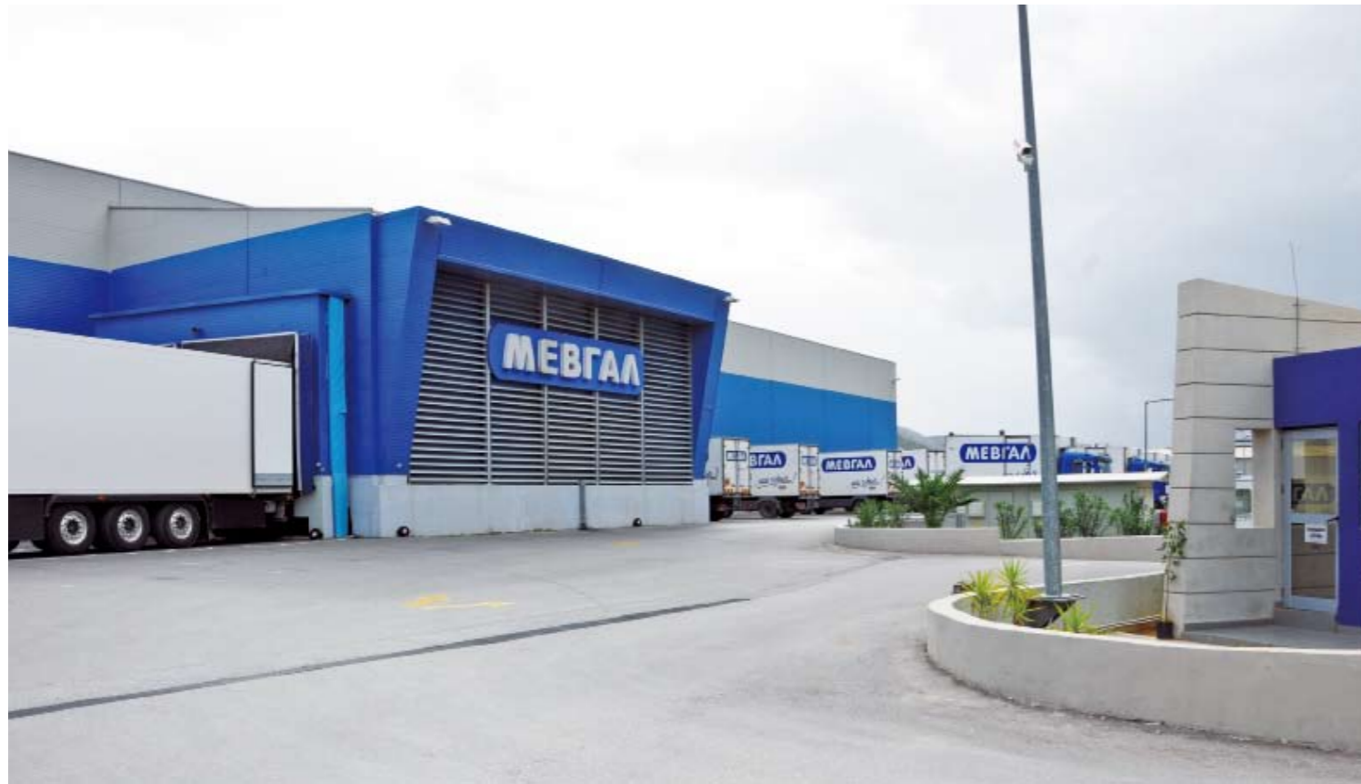
A view of the warehouse cargo unloading area
