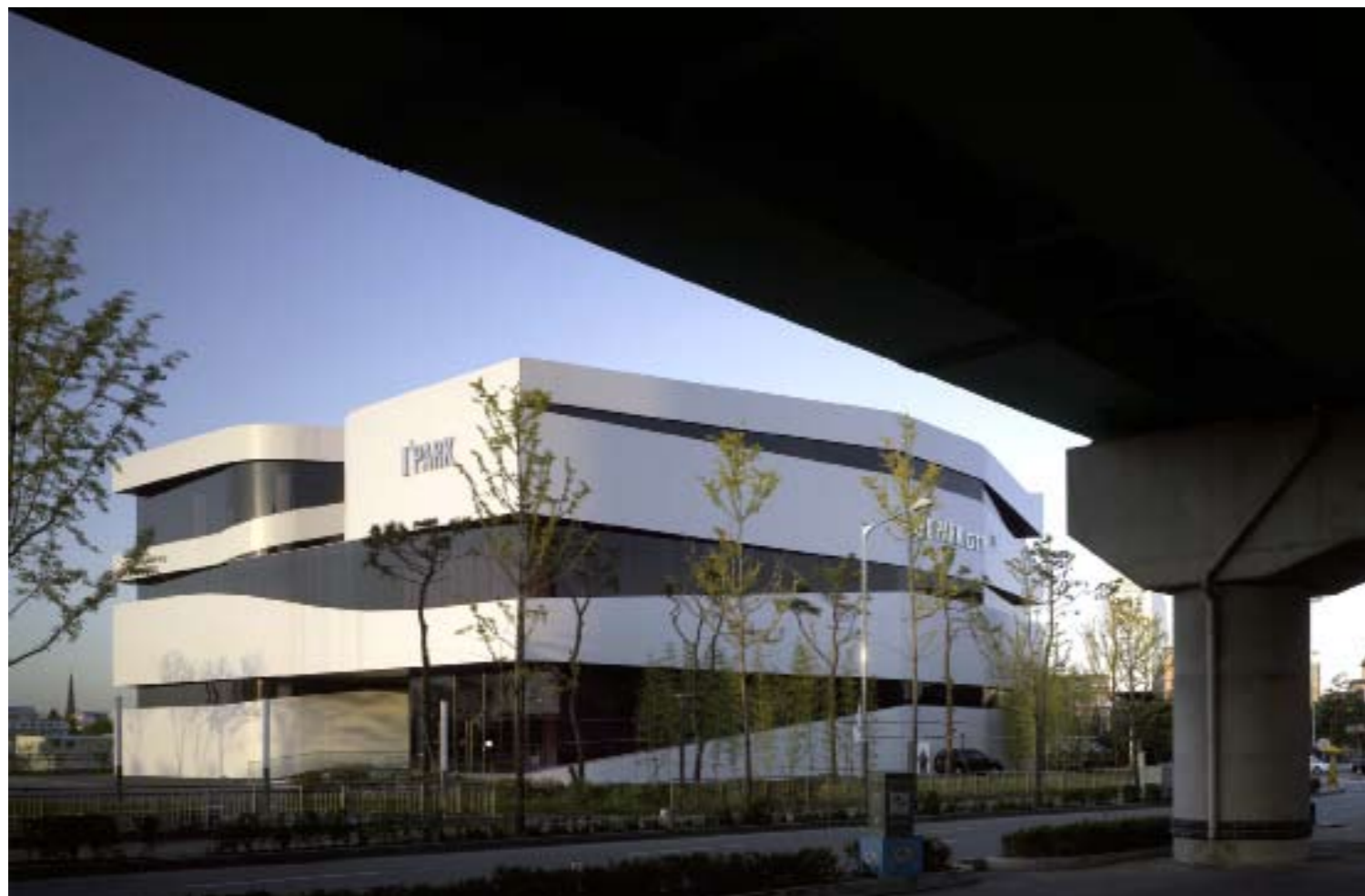
Building in normal environment
