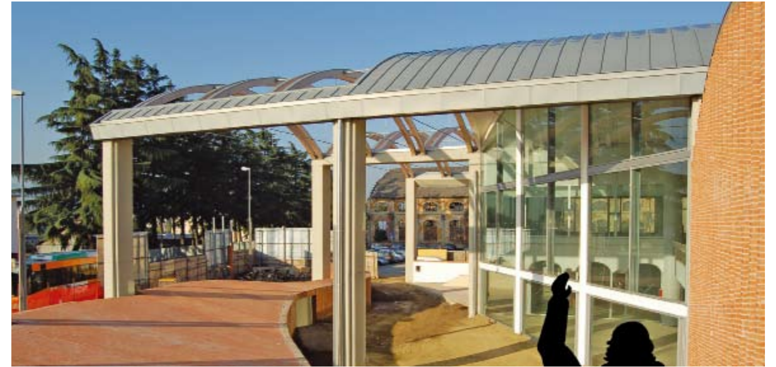
Architectural relation between the library and the water and power plant
