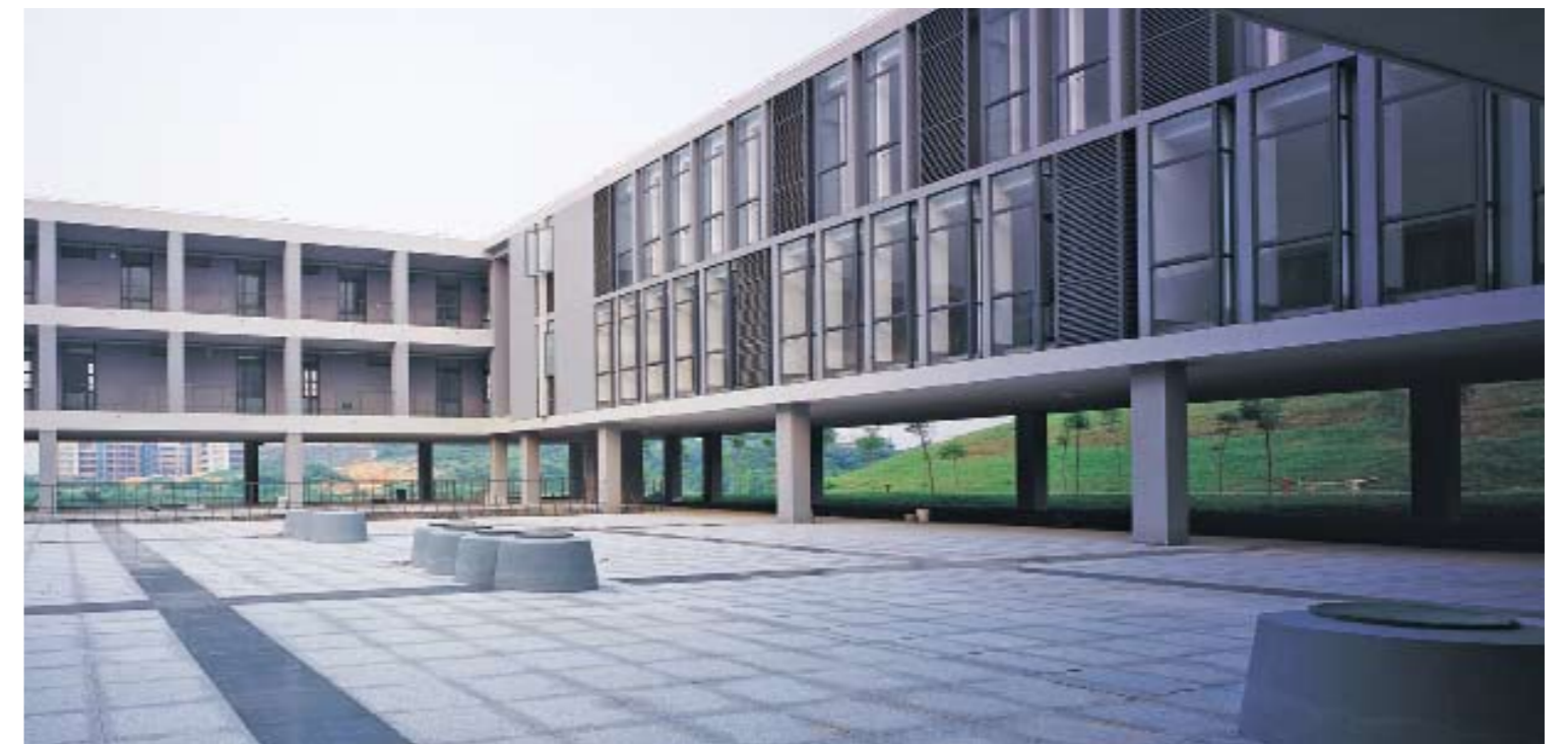
Inner court of the 2nd floor
