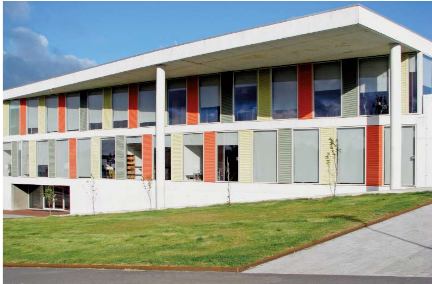
Stepped ramp and canopy on south side
