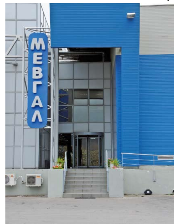
A view of the office building facility entrance 02
