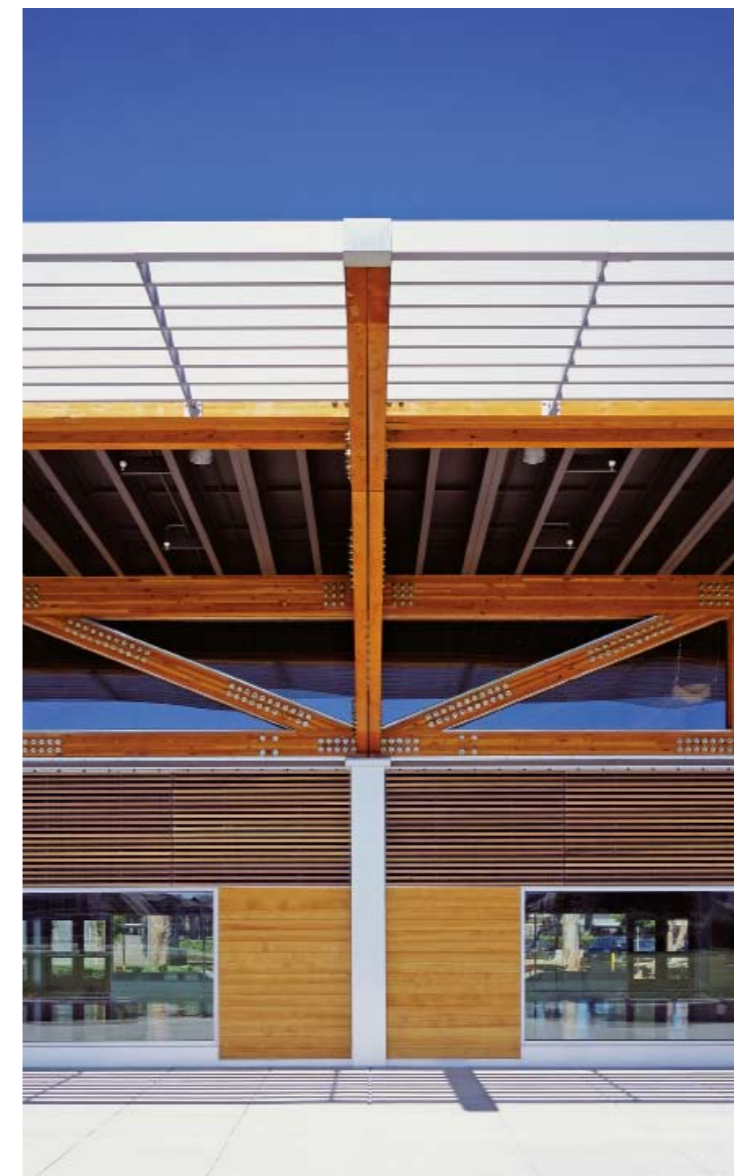
Detailed exterior cedar and glass façade of multi-purpose pavilion on west, south and east sides
