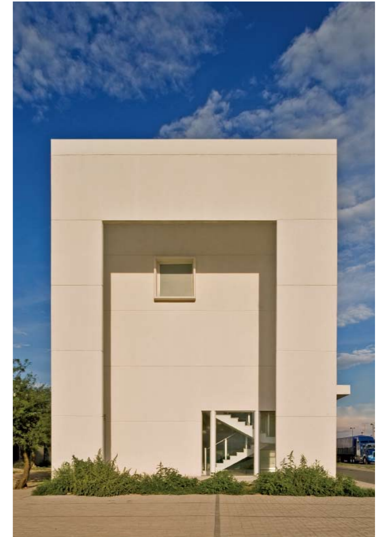
The long and slim terrain, facing one of the main avenues in the city, dictated the programme
