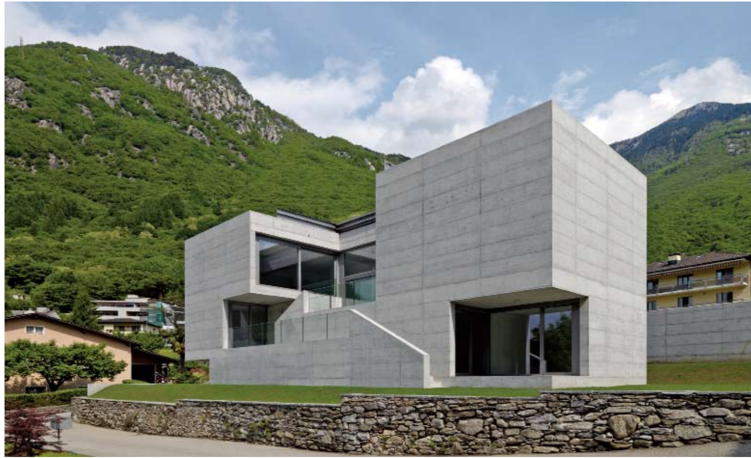
External view of the house in its Alpine context from the southeast
