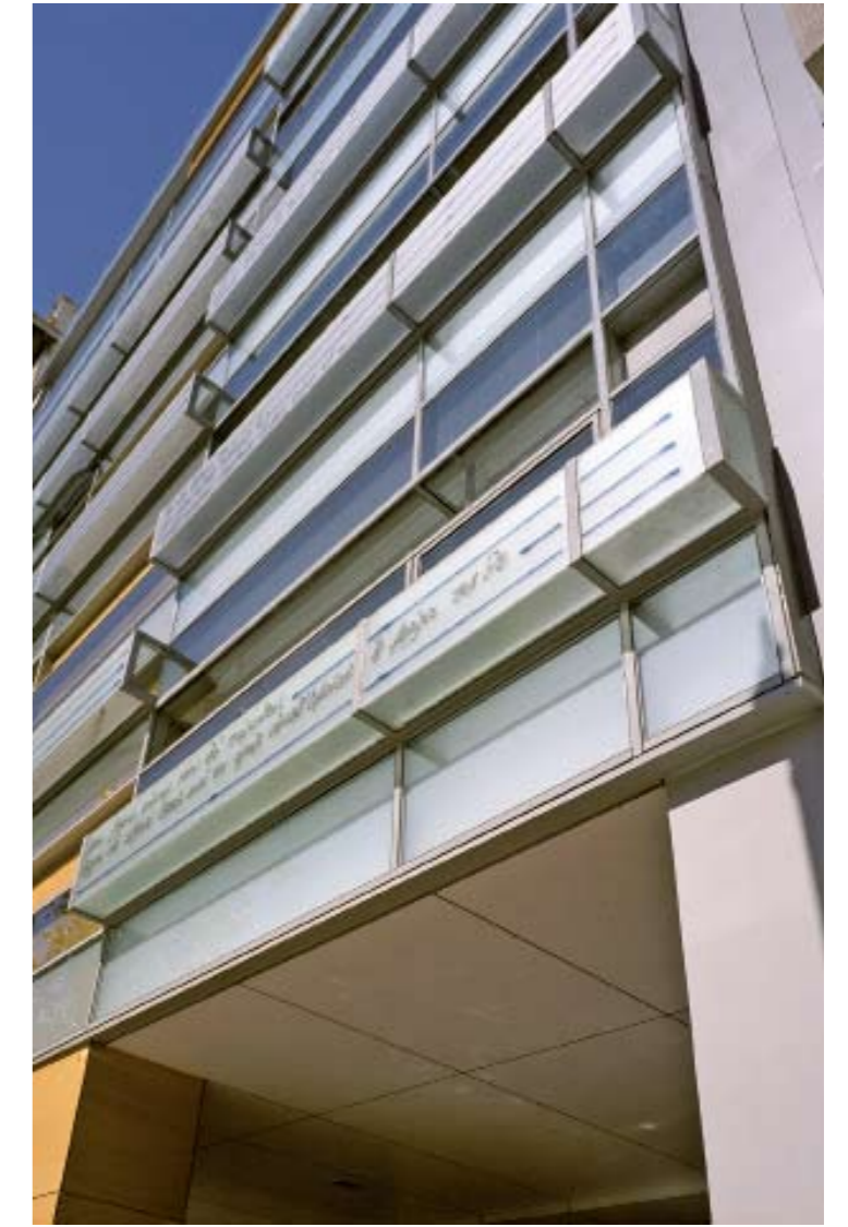
Details of façade
