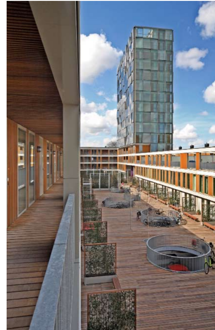
Courtyard on the roof
