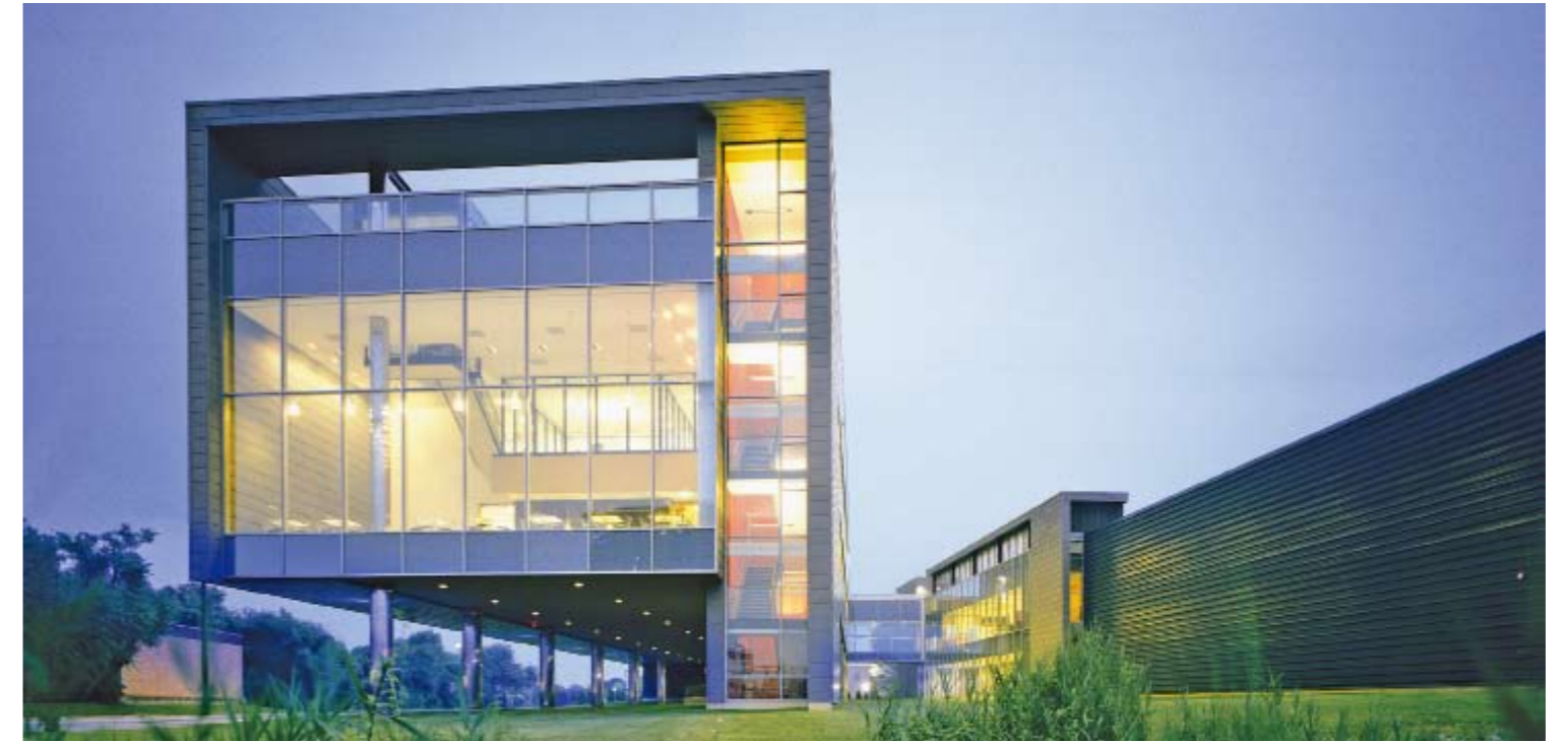
View from west towards office building common area and terrace
