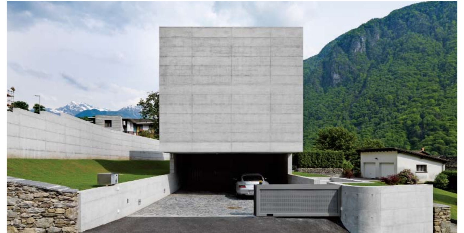
View from west to parking and entrance
