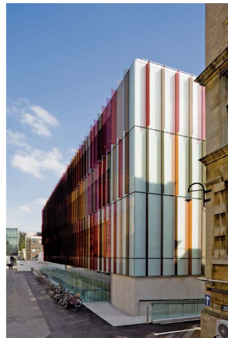
Coloured glass fins fixed vertically within the mullions wrap the full perimeter of the building
