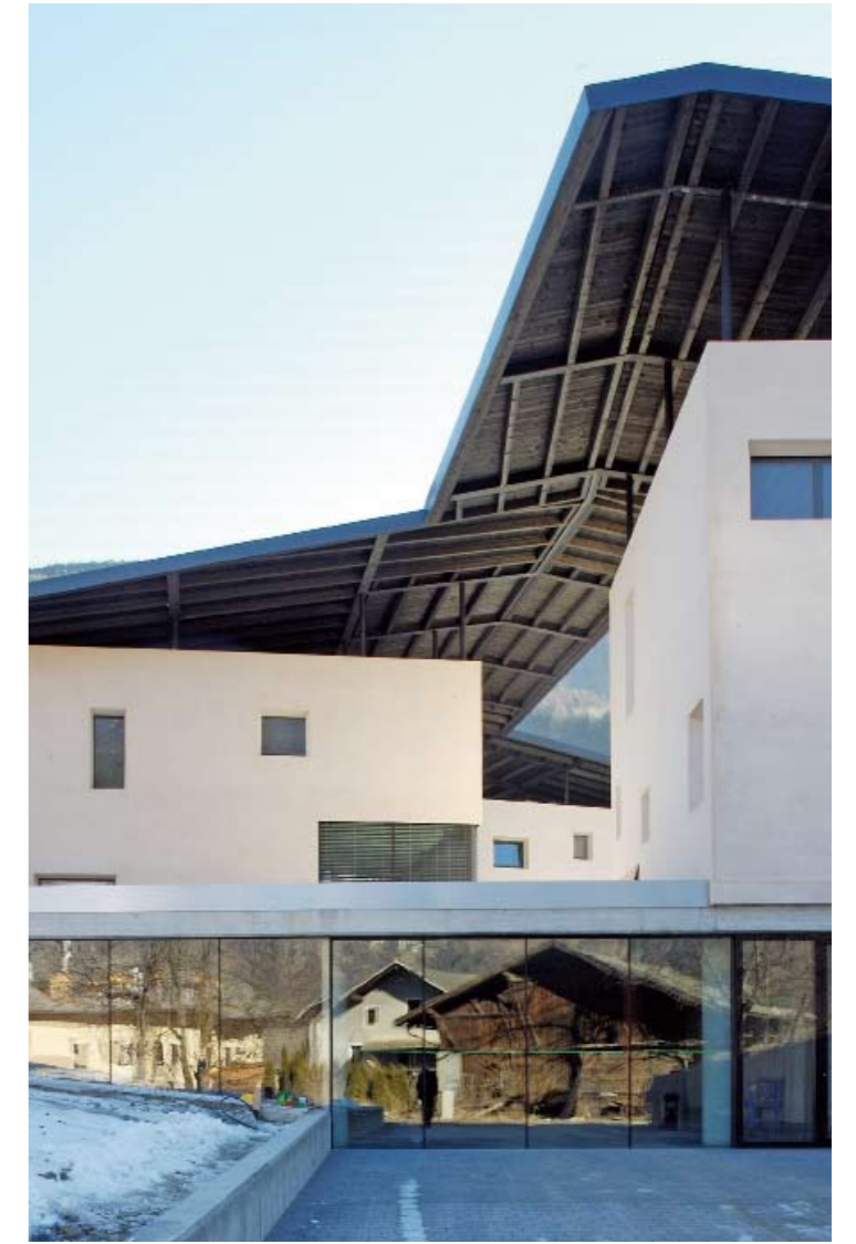
Side view of the exterior
