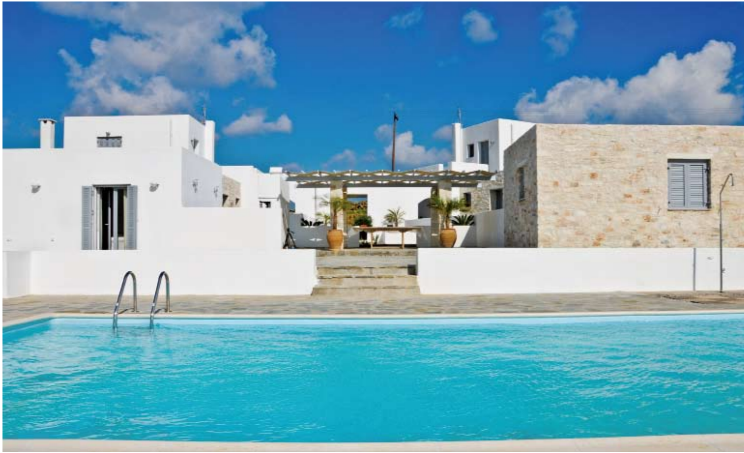
A view of the stairwell leading to the swimming pool from the main yard
