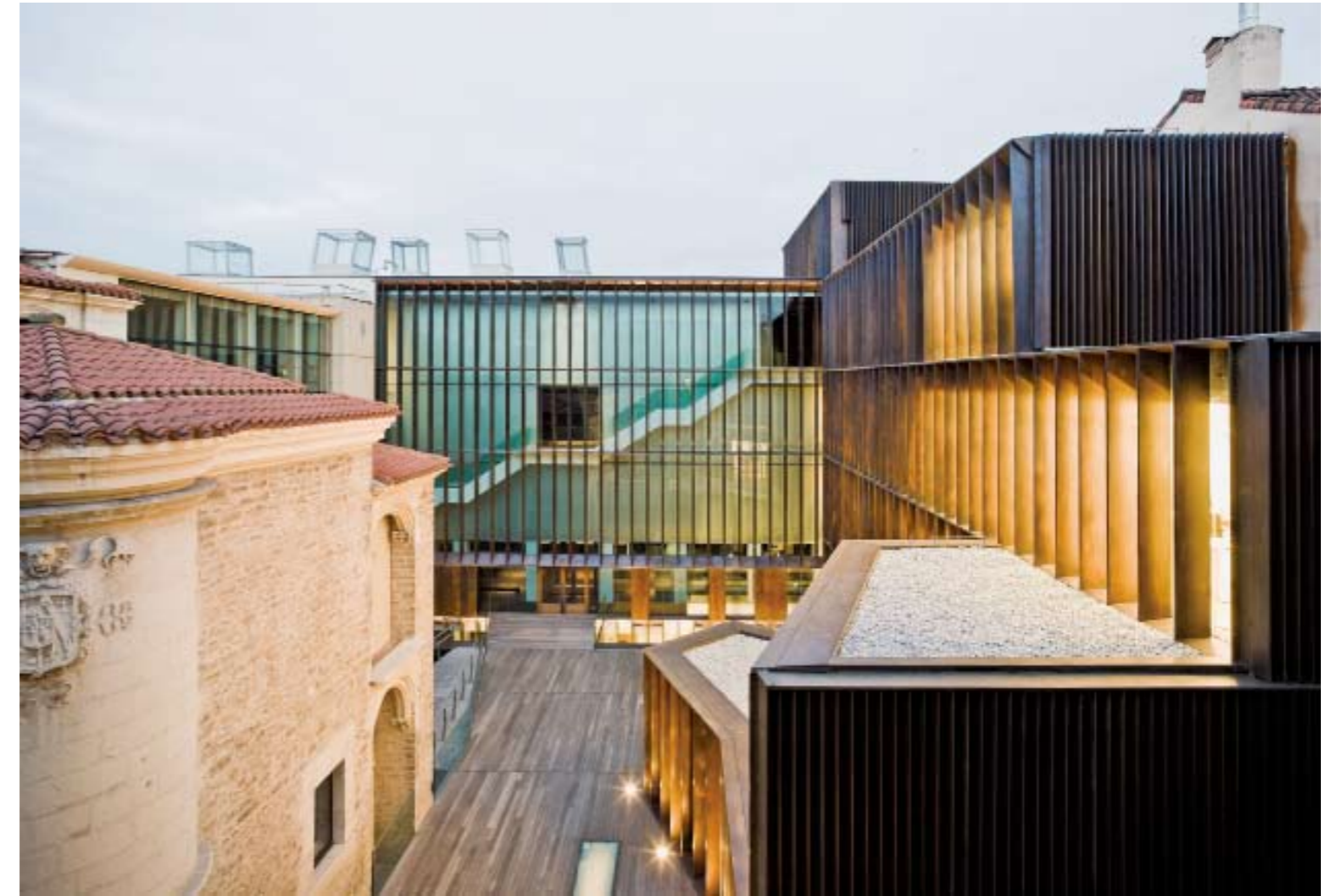
Cast bronze pieces configure the outer façades that define the access court
