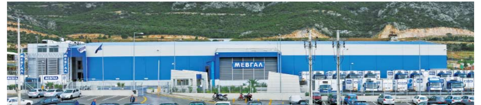
A general view of the entire complex: warehouse, cold storage, and office facilities
