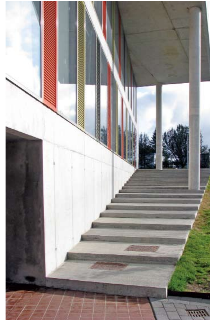
Stepped ramp and canopy on south side
