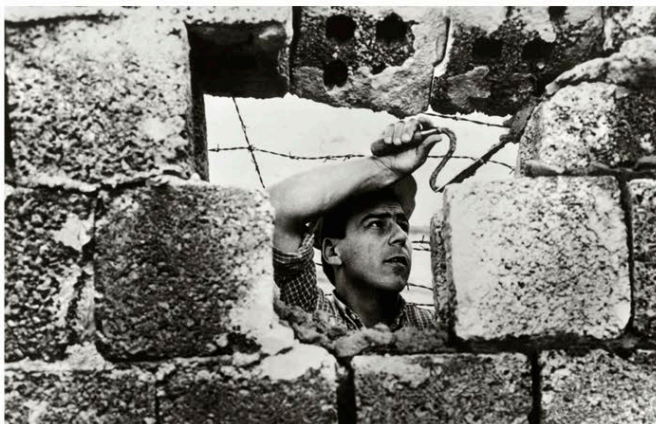
◁ Concrete divide An East German worker makes repairs to the hastily built Berlin Wall—a 28-mile (45-km) scar that cut through the German capital, dividing east from west.
