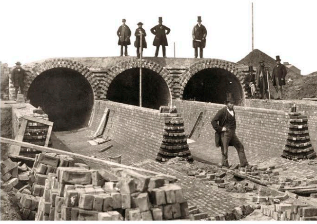
◁ Cleaning up British engineer Sir Joseph William Bazalgette (top right) surveys work on London's sewers. His sanitation systems transformed public health in cities around the world.
