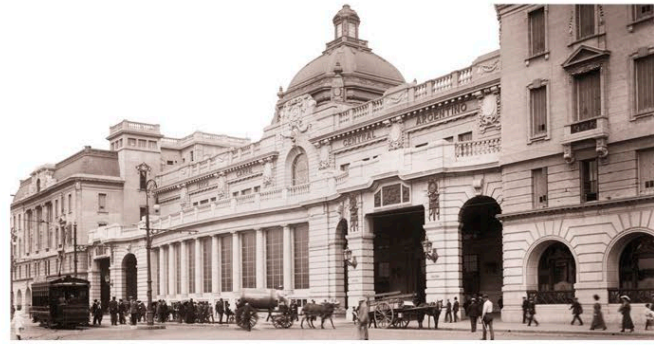
◁ Soft imperialism Built with British expertise, using British materials, the Retiro Railway Station in Buenos Aires is an example of how imperial influence extended beyond official colonies through cultural, financial, and industrial means.
