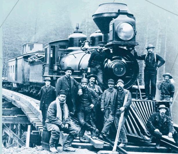
△ Railroad construction crew
