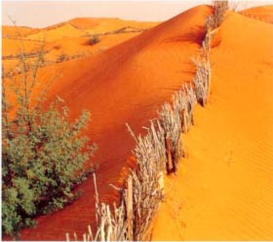
**In Mauritania the Fightthe Desert project uses simple strategies to prevent the spread of the desert. Fences of wood from a local tree are placed in 30-by-30 meter (98×98 foot) squares to prevent the sand from blowing away, there by stabilizing the desert soil.**
