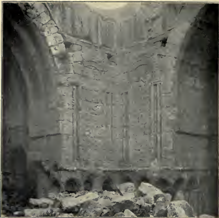
29 Ammān, square building with apse-buttresses ; blind arcade with formal ornament. See pp. 123, 124.
