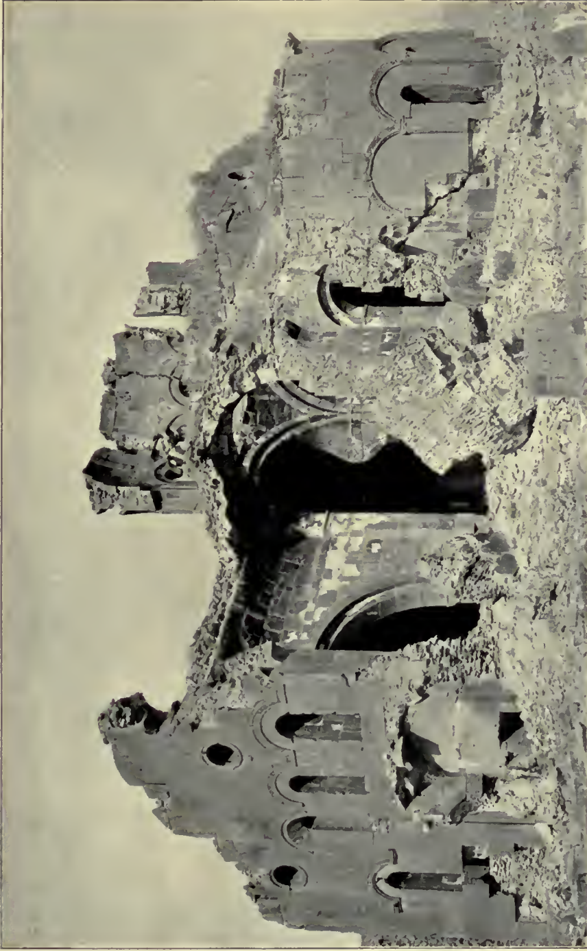
10 Thalin, cathedral, sixth-seventh century, from South-West ; three-aisled trefoil-ended type ; the dome fallen in. See pp. 70, 214.
