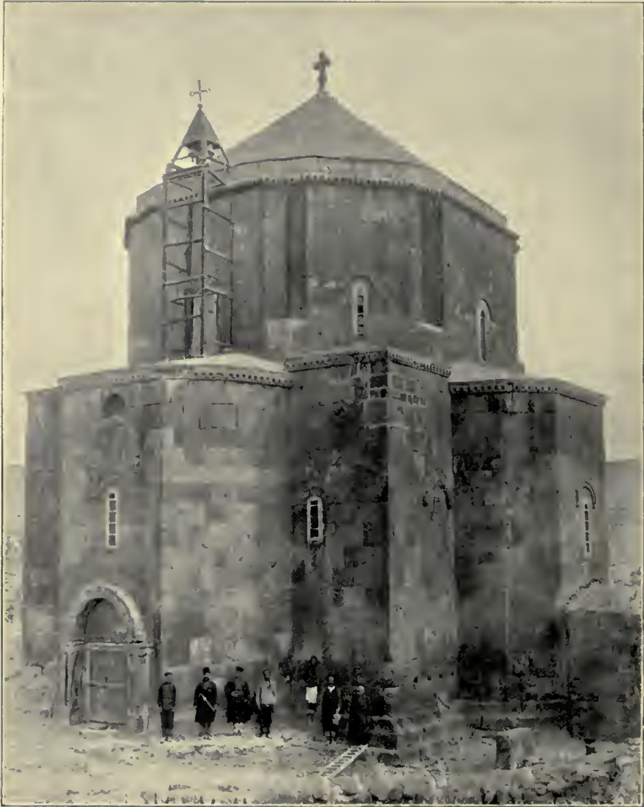
1 Maštara, domed square with apse-buttresses, c. A.D. 650 ; exterior from South-West. See p. 61.
