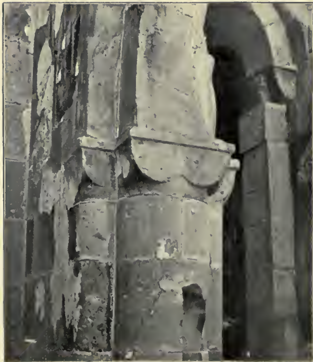
24 Thalin, cathedral ; detail of South-West pier. See pp. 95, 145, 146.
