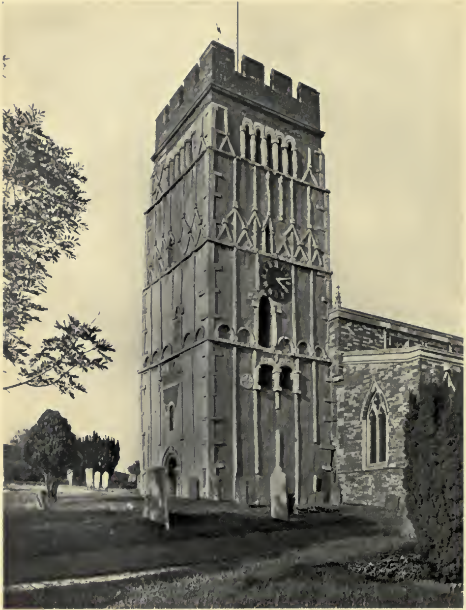
Earls Barton Tower, Northamptonshire.
