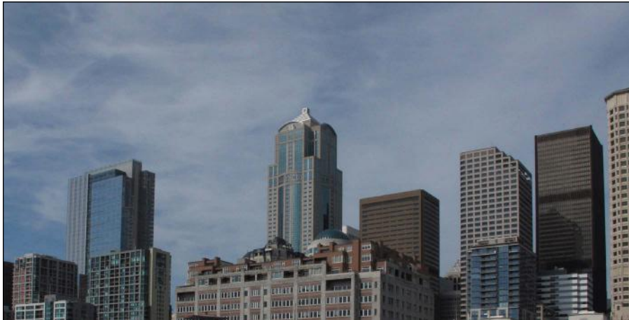
Figure 11-8: The corrected tower looks like this.
