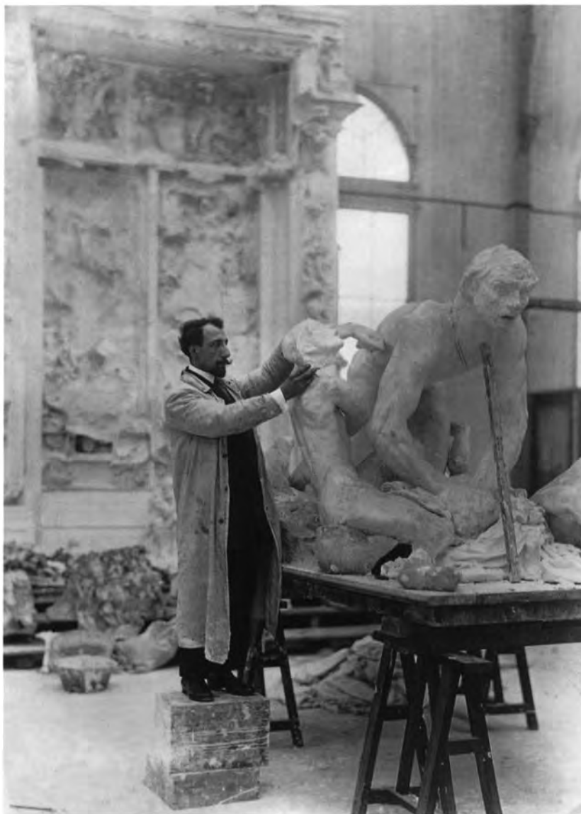
far left: Fig. 12. Three views of sculpture technician Georges Bigel in his Paris studio using a Collas machine to reproduce a sculpture.
