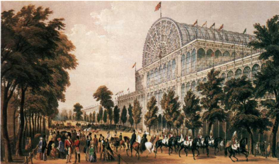
Paxton, The Crystal Palace, 1850-51, (destroyed by fire, 1935), Guildhall Library, London. The Crystal Palace was the first iron-and-glass structure built on such a huge scale that showed industrial materials were both functional and beautiful.
