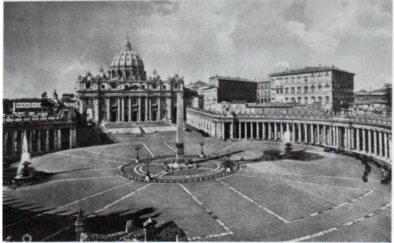
Aerial view of the piazza, St. Peter's Cathedral, Rome.
