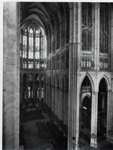
Choir of Beauvais Cathedral , begun 1272. Beauvais Cathedral's linear design and pointed arches are characteristic of Gothic architecture.
