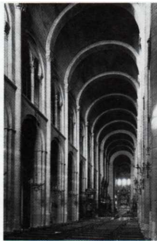
The nave of St. Sernin showing barrel vaults, c. 1080–1120.
