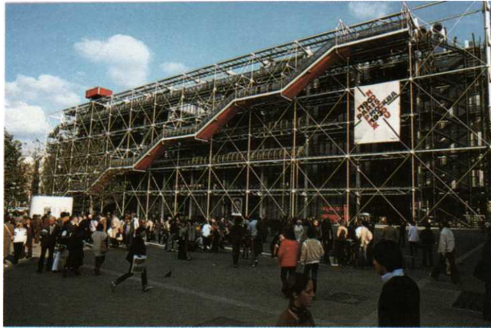
Piano and Rogers, Centre Pompidou, 1977, Paris. This building celebrates technology by putting beams, ductwork, pipes, and corridors on the outside.
