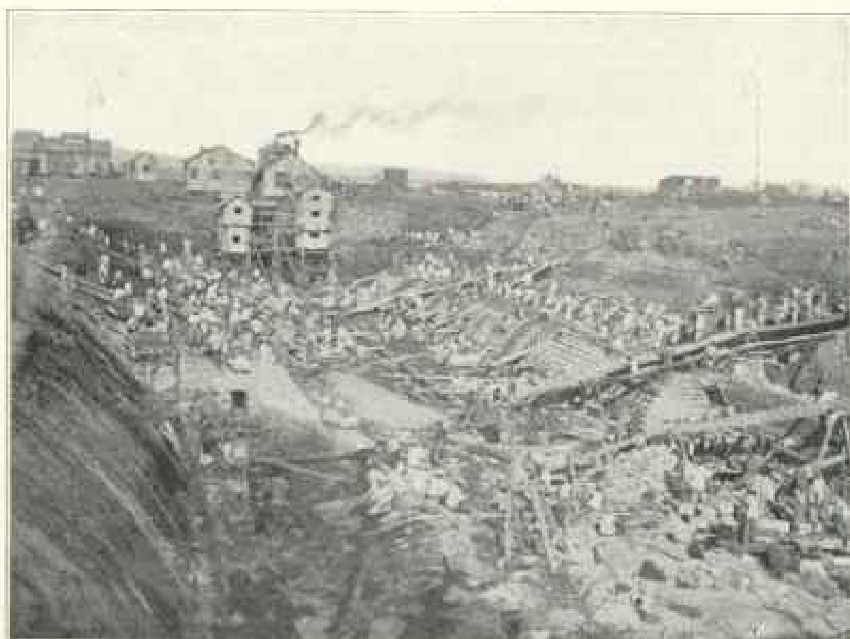
Constructing a Dry Dock at Dalny
