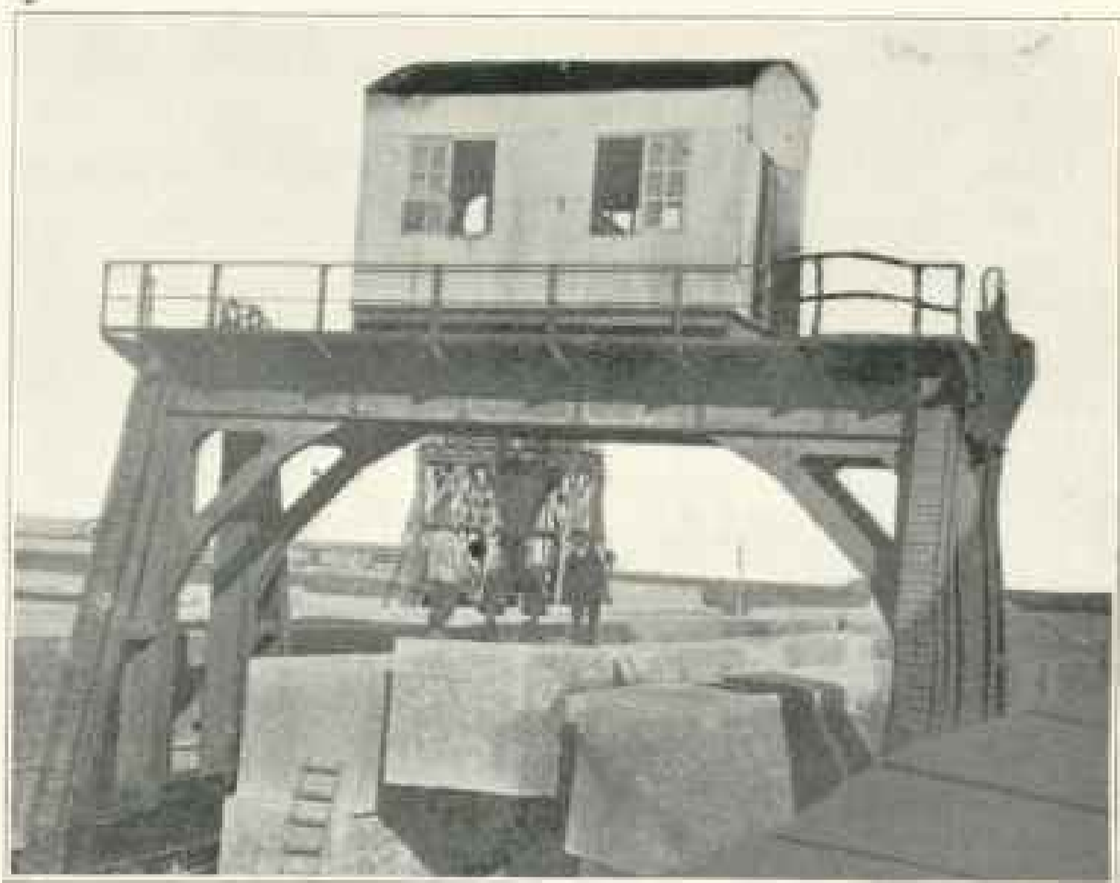
Handling the 50-ton Blocks for Construction of Piers, Dalny
