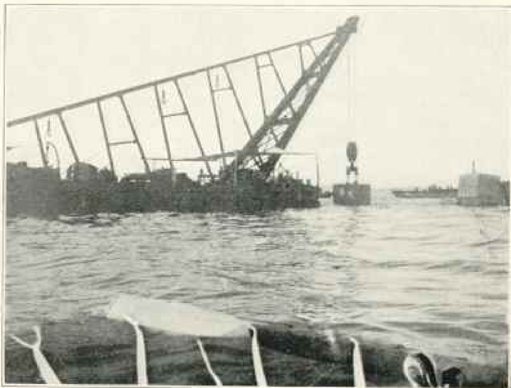
Laying the 50-ton Blocks for the Piers, Dalny
