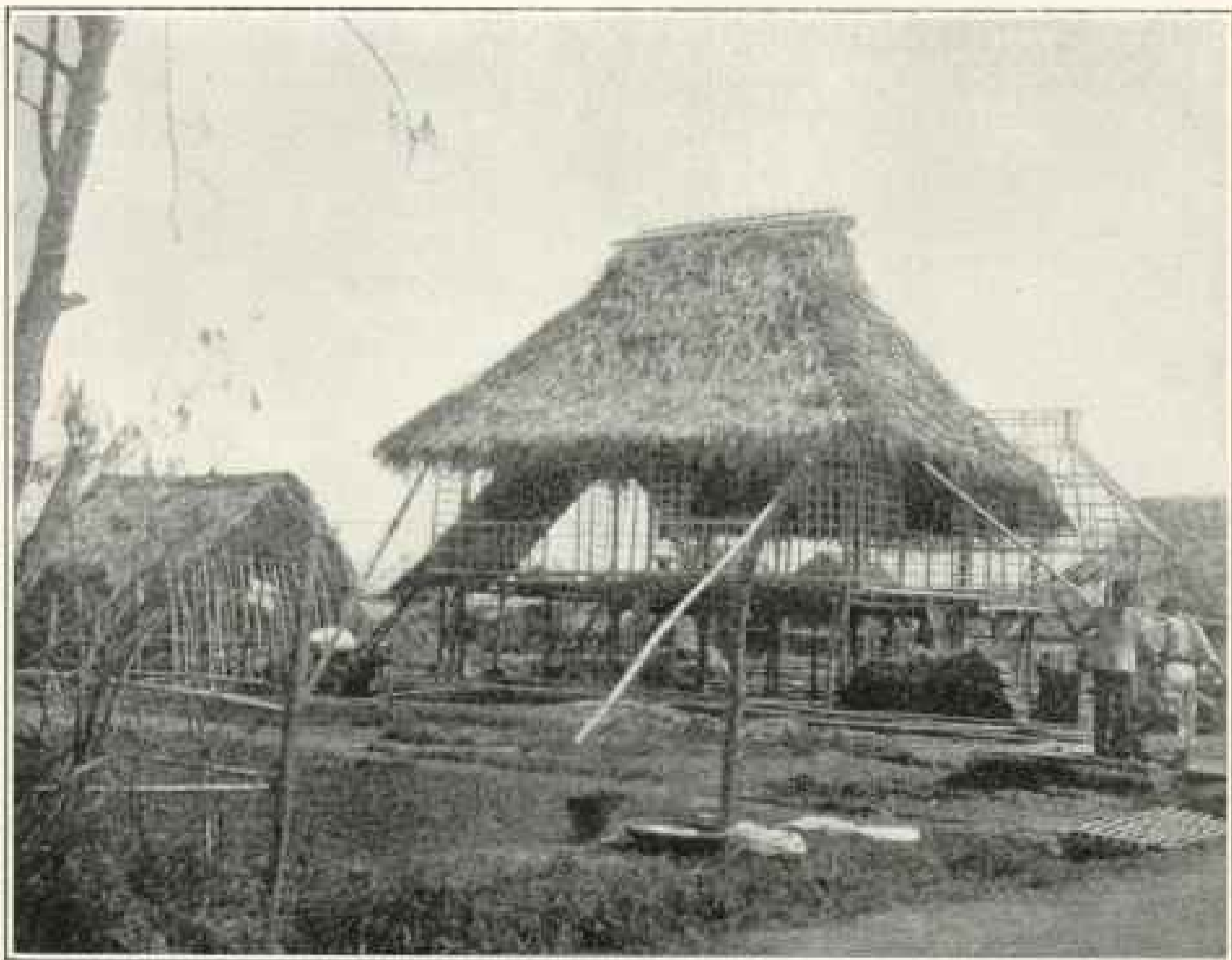
Nipa House Under Construction
