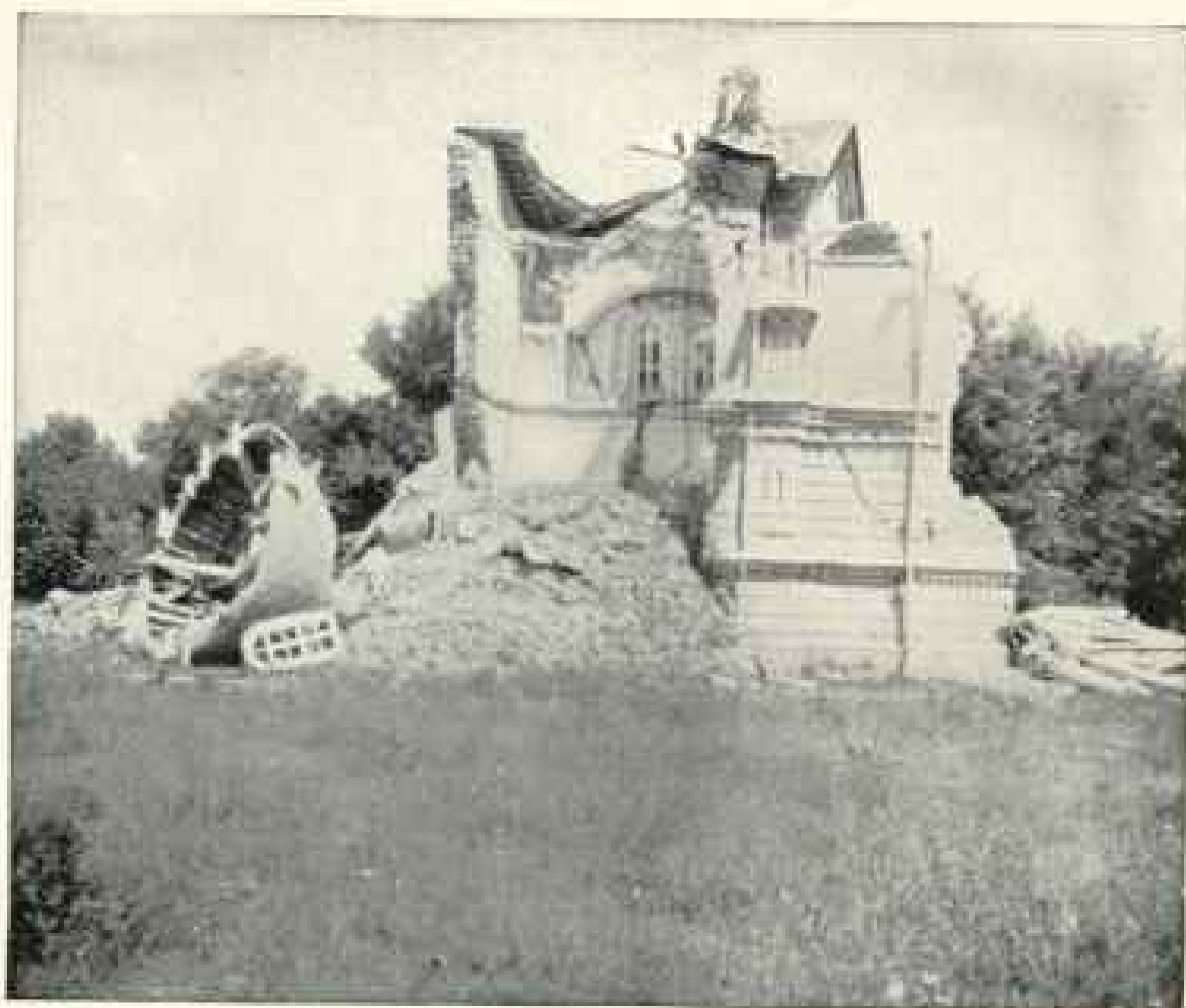
Russian Chapel after the Earthquake, Andijan
