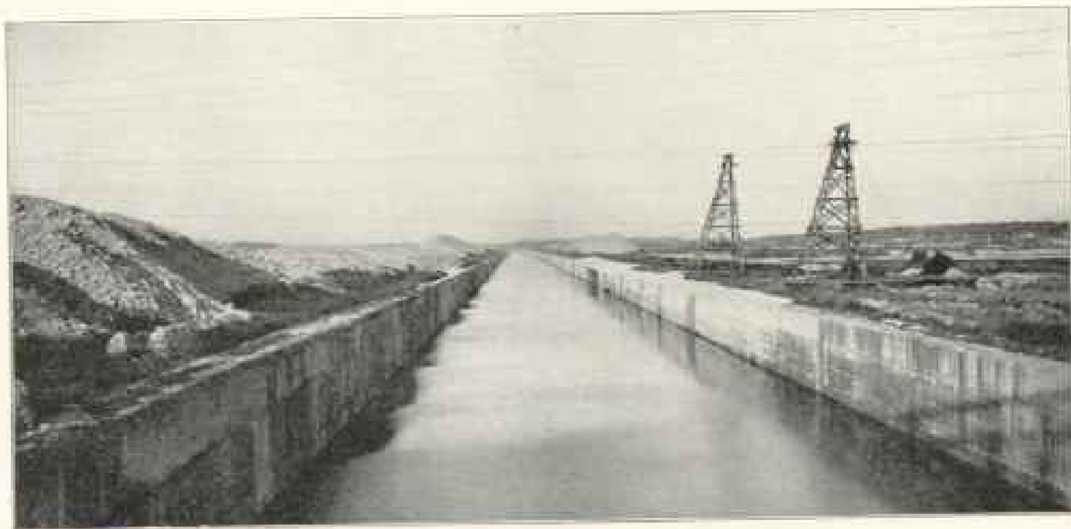
A View of the Chicago Drainage Canal
