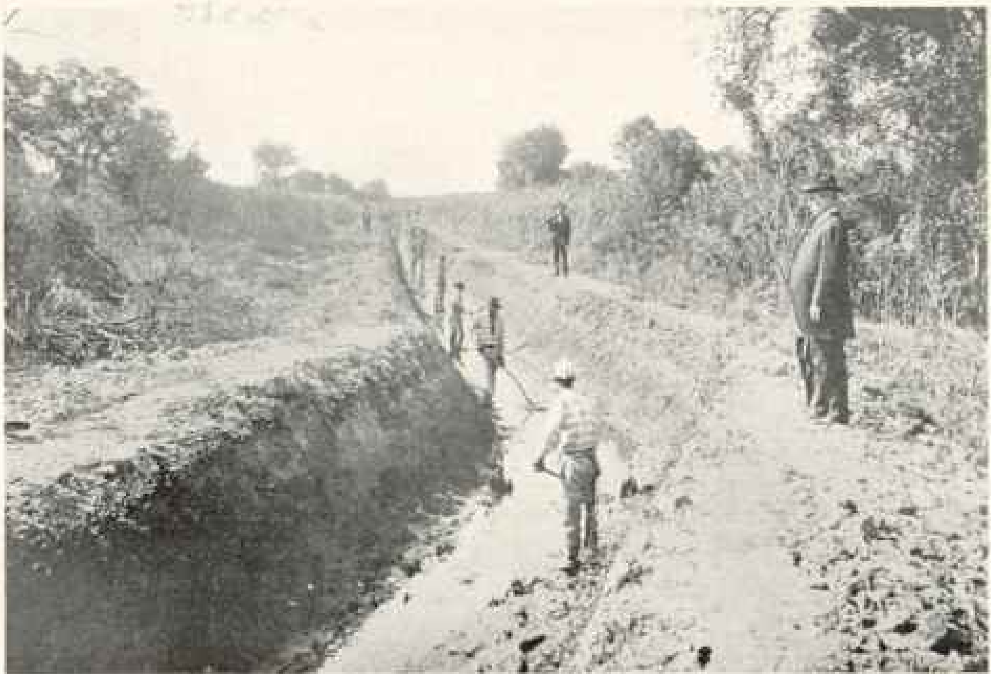
MINNESOTA SWAMP SURVEY (U. S. GEOLOGICAL SURVEY PARTY EN ROUTE) HAND-DITCHING BY CONTRACT LABOR, HOLBECK'S SWAMP, NEAR CHARLESTON, S. C.
