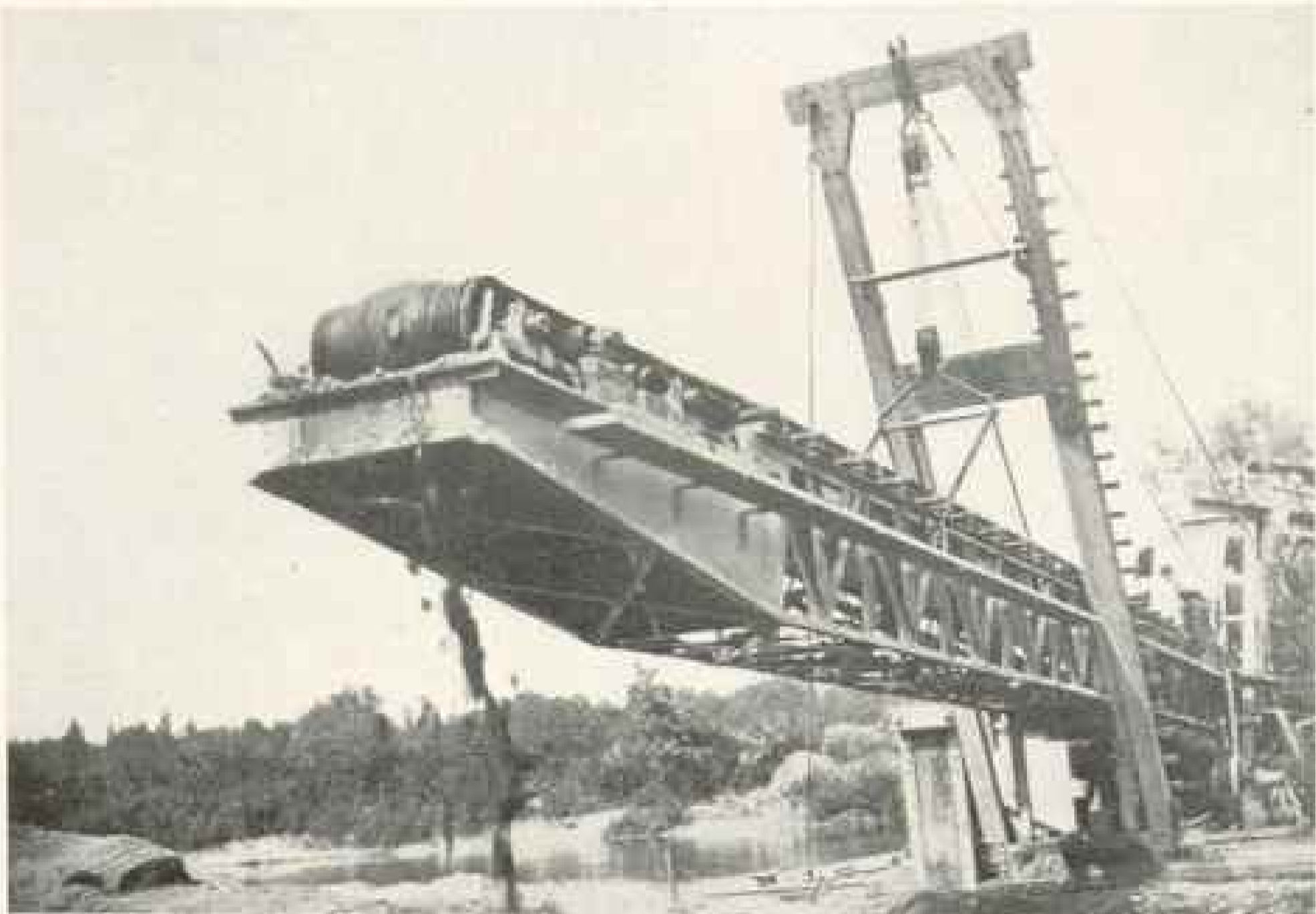
TYPE OF CONVEYOR DREDGE USED IN CHANNEL-DEEPENING
