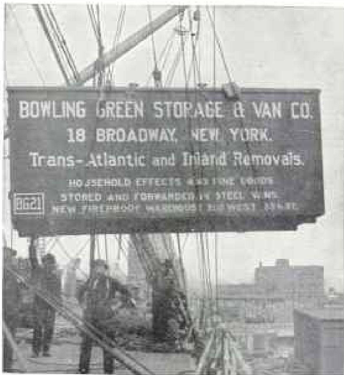
HOISTING LIFT-VAN ON BOARD STEAMSHIP
