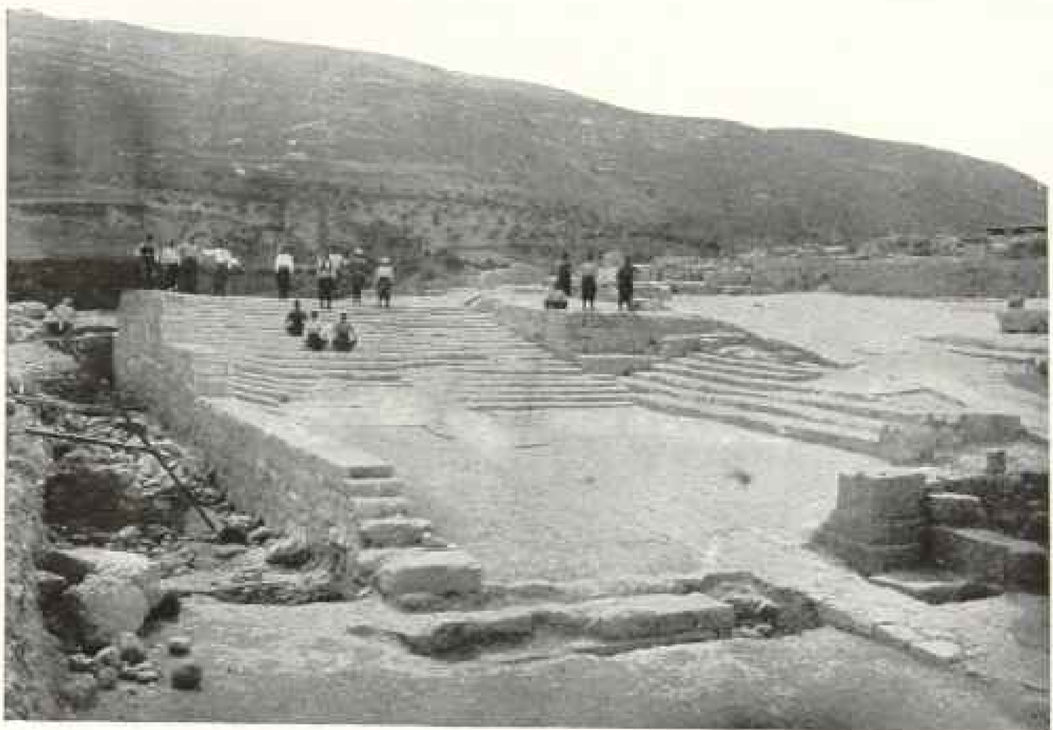
THEATRICAL AREA, KNOSSOS, RESTORED (NEAR MODERN CANDIA)
