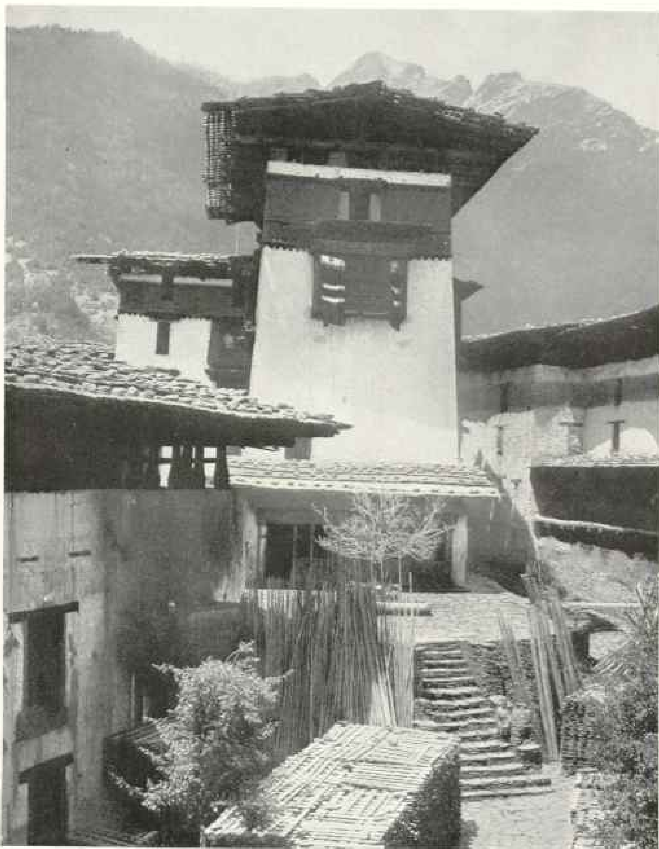
A VIEW OF THE INTERIOR OF DUG-GYE JONG, SHOWING SHINGLE ROOFS KEPT IN PLACE BY LARGE STONES
