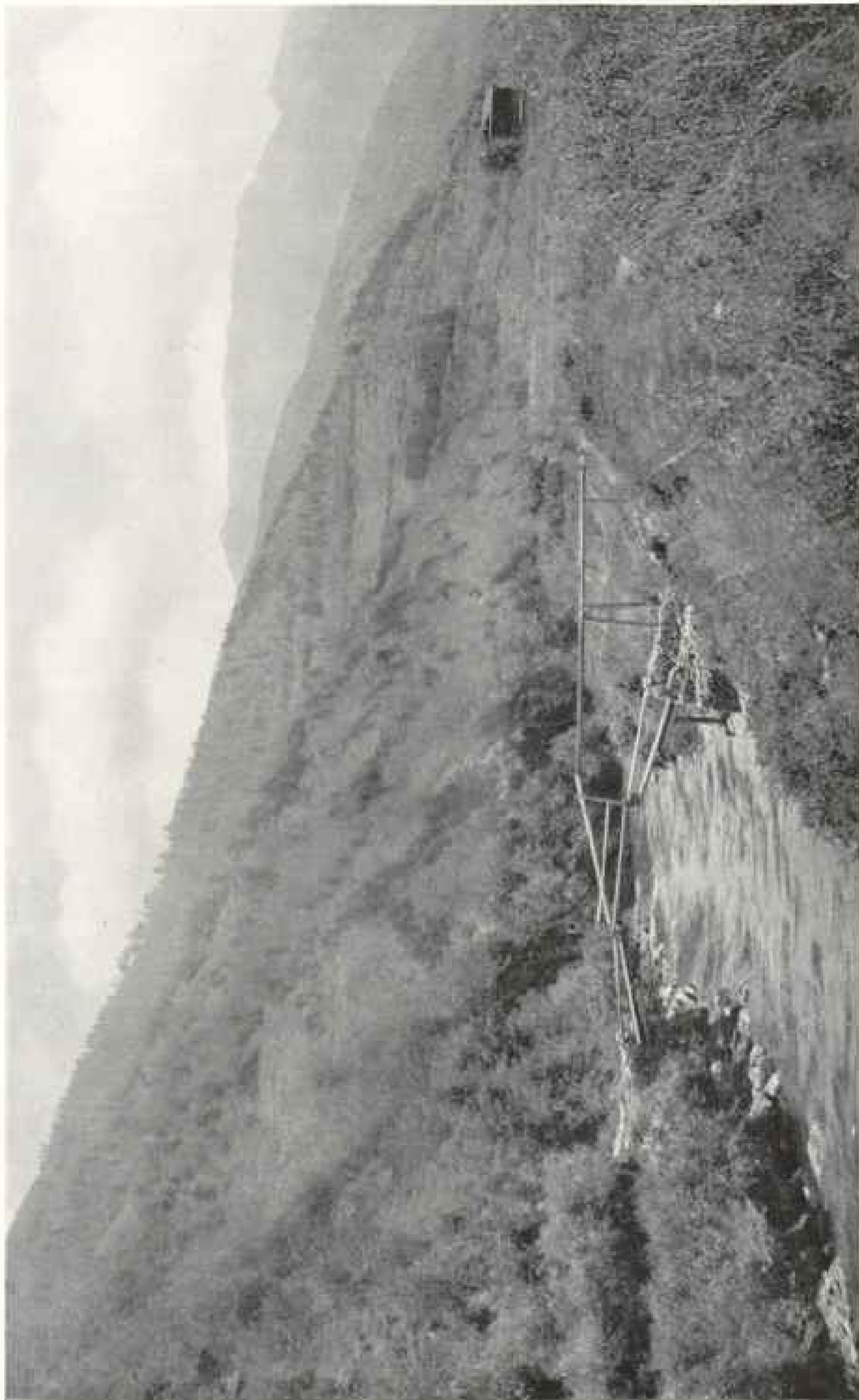
METHOD OF CARRYING WATER ACROSS A RIVER FOR IRRIGATION PURPOSES BY MEANS OF HOLLOWED-OUT TREE TRUNKS
