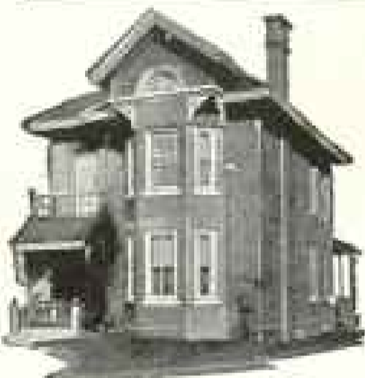
A Big House in a Cold Part of Canada
