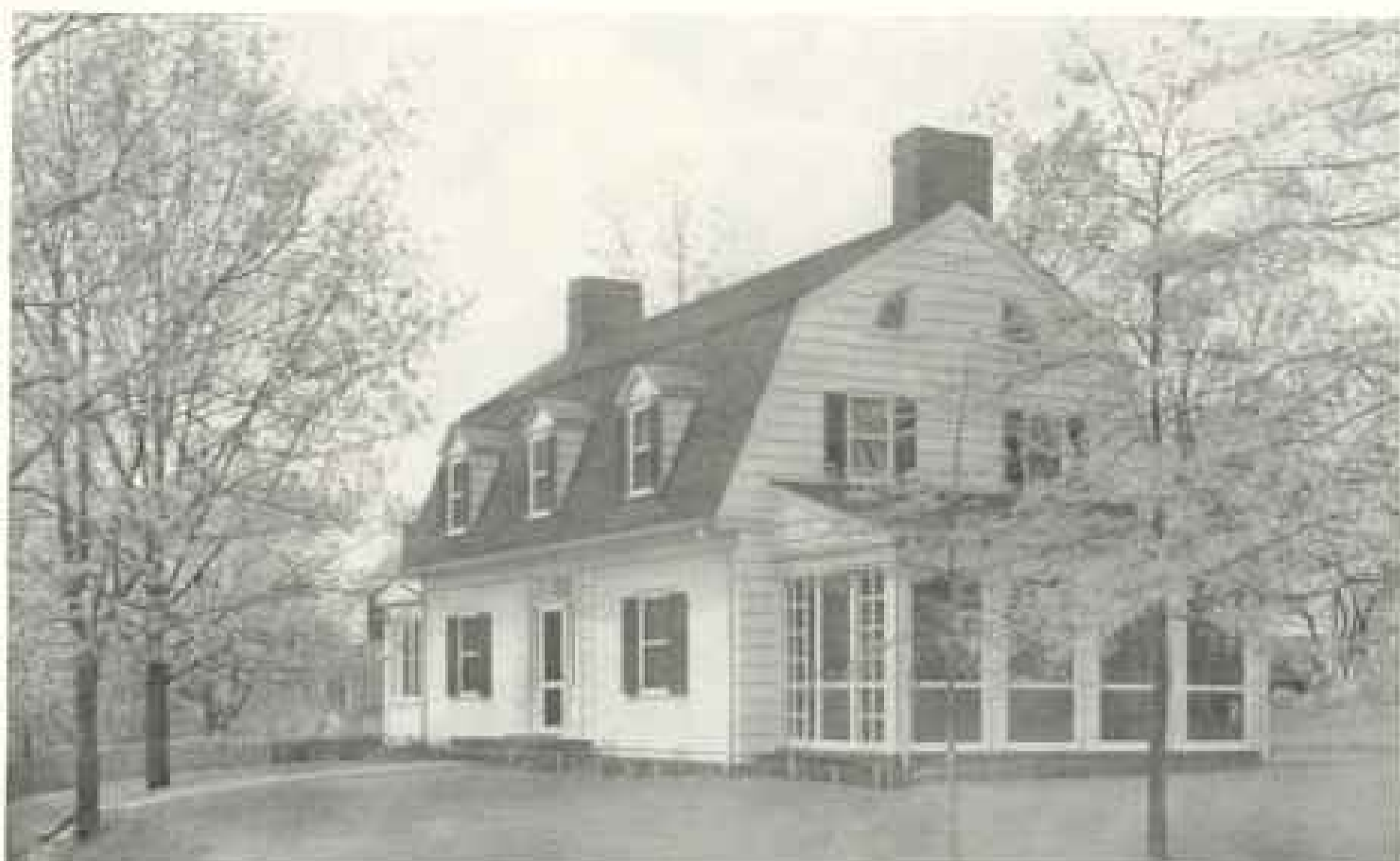
House of Daniel W. Nye, Esq., Katz Gardens, Long Island, N. Y. Aymar Embury II, Architect, New York, N. Y.
