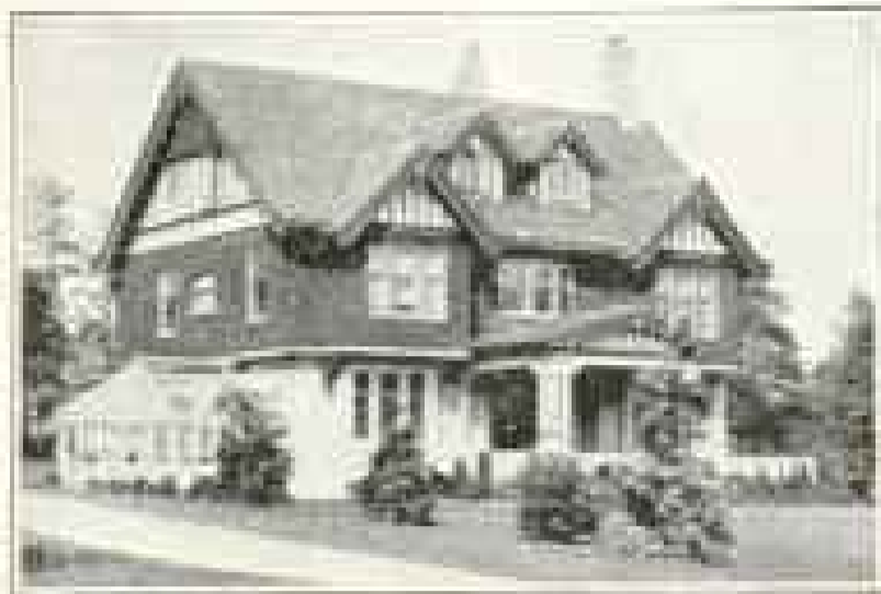
RESIDENCE OF CHARLES MORSE, JOHNSTON BL., CINCINNATI, OHIO. E. H. BARNETT, ARCHITECT
