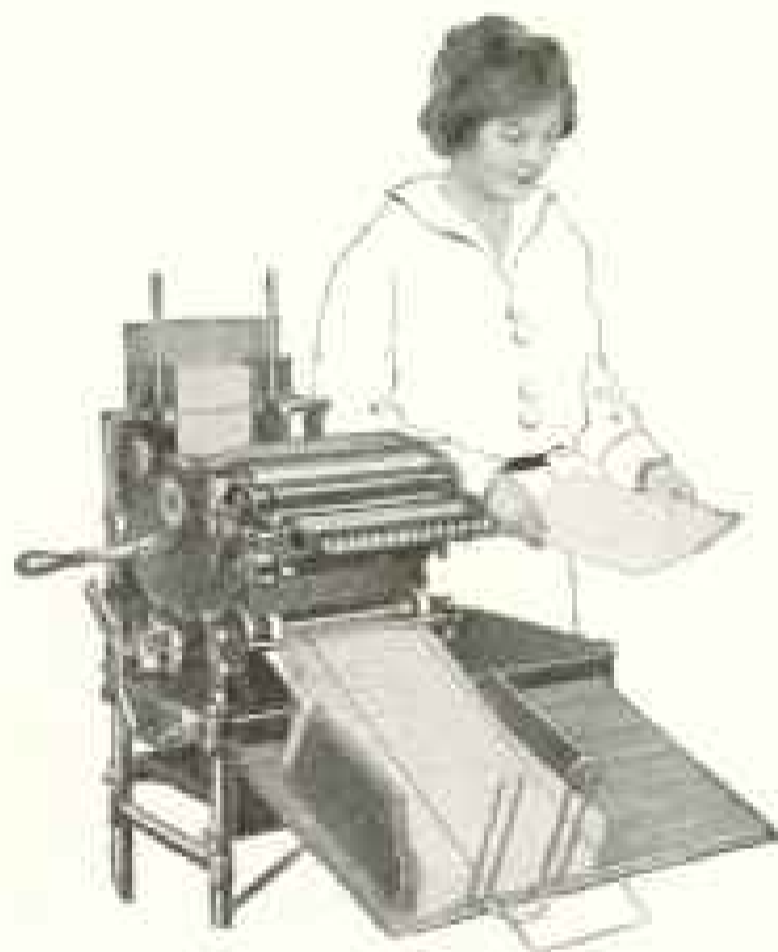
Multigraph Senior—Electrically driven and completely equipped for high-grade printing with printers' ink, type or electrotype, or for producing typewritten letters in quantities. Prices, $670 to $720. Hand-driven models, $280 up. Easy payments.
