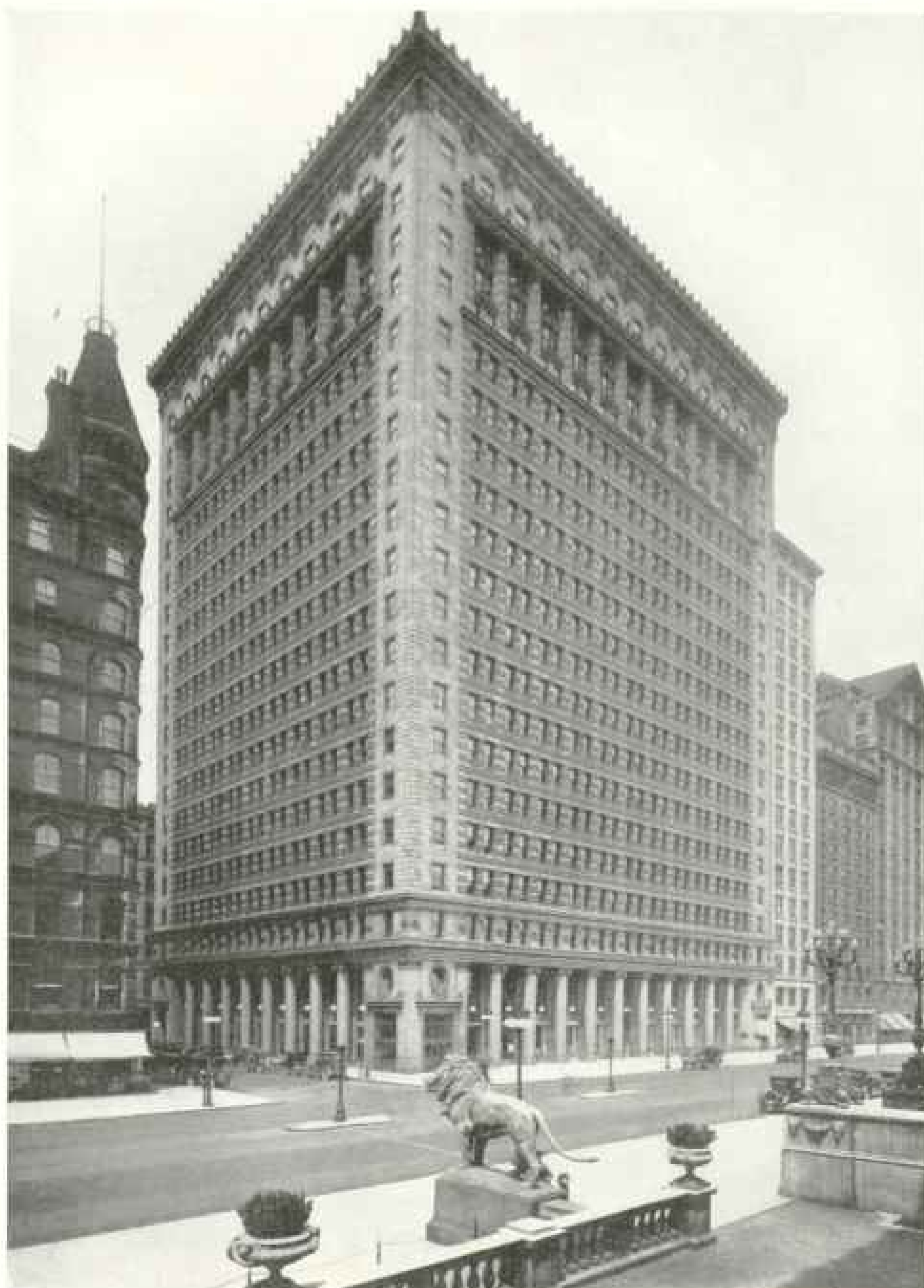
Photograph from Chicago Architectural Photo Company
