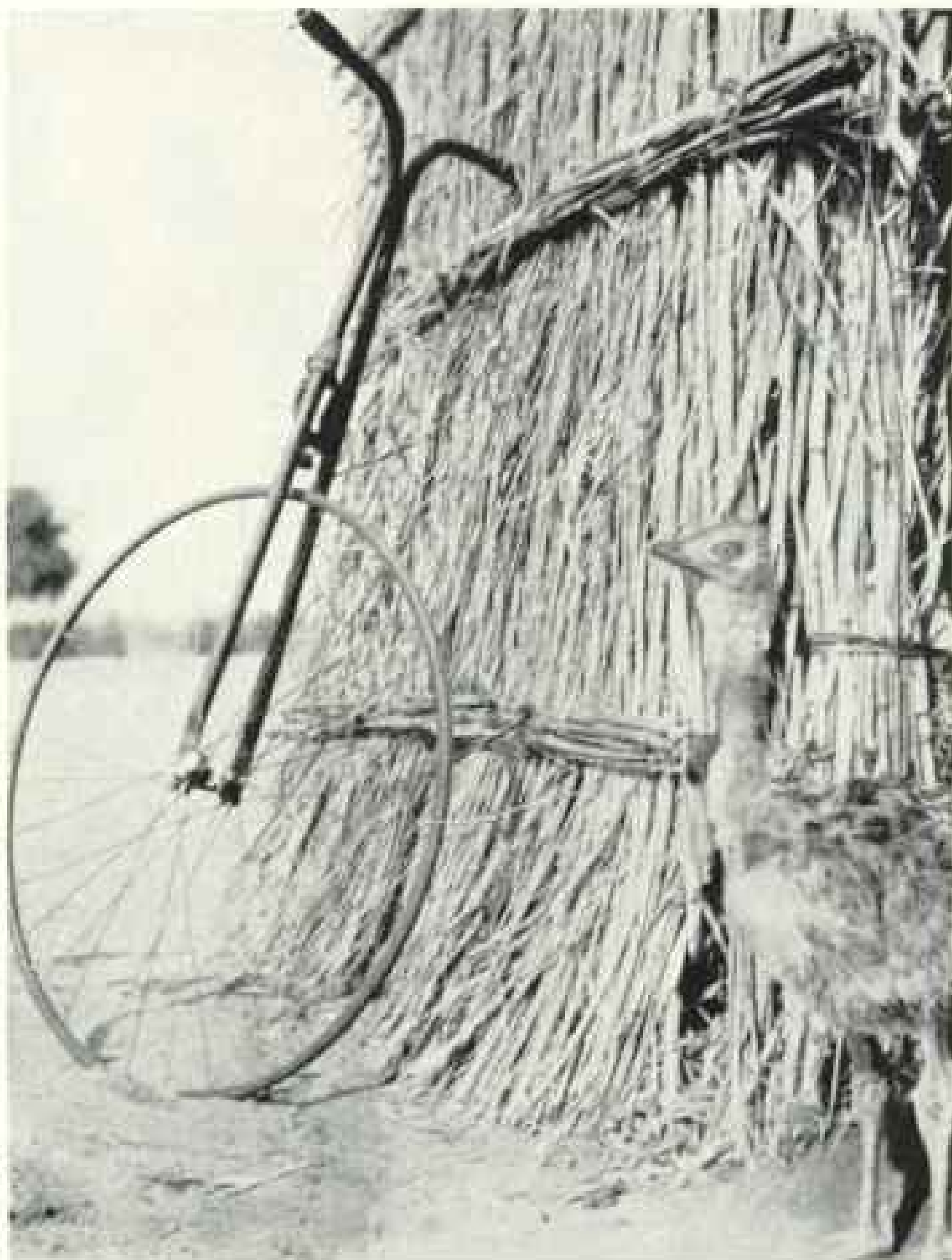
THE SURVEY WHEEL USED BY THE AUTHOR IN MAPPING DARFUR
