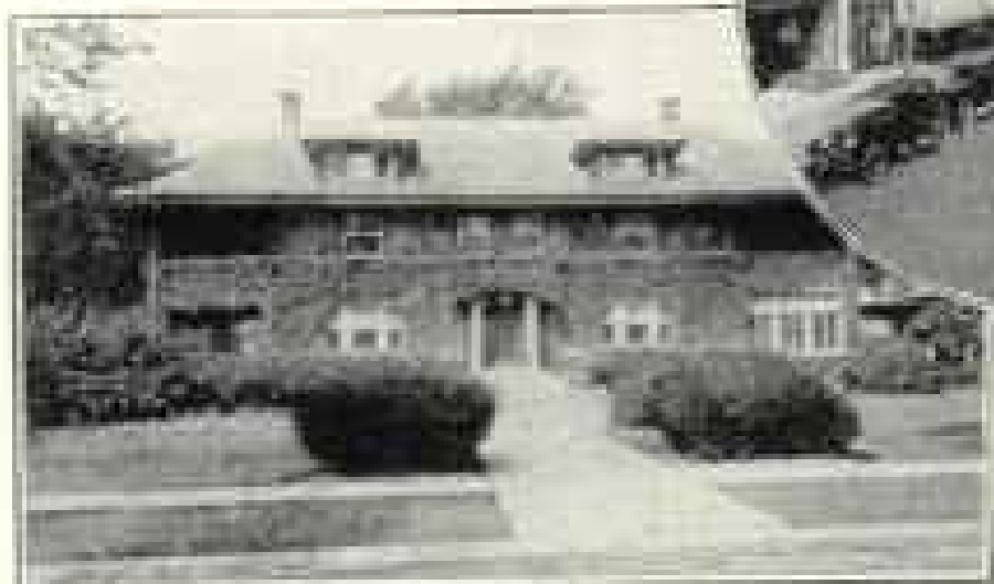
Typical of the homes that grace Oak Park, is this lovely place on Euclid Ave. In the circle above are shown six shops on Martin Street heated by Oil-O-Matic
