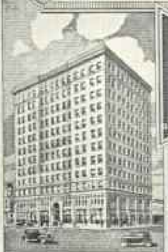
VOLUNTEER STATE LIFE BUILDING CHATTANOOGA, TENN. ARCHITECT—BARNARD W. BARNETT CONTRACTOR—W. B. WAIN
