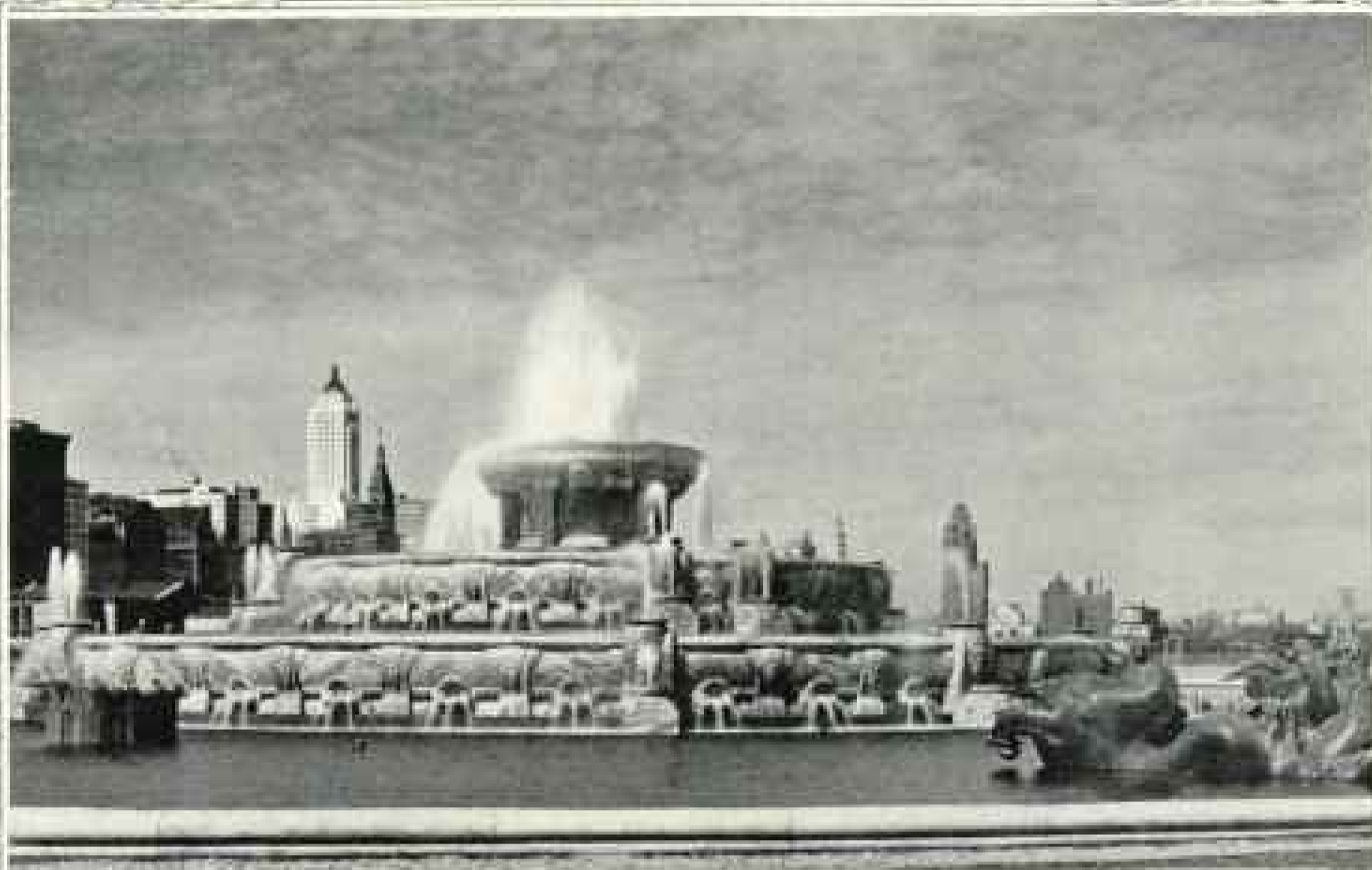
BUCKINGHAM MEMORIAL FOUNTAIN CHICAGO DENNET, PARSONS & FRUST ARCHITECTS
