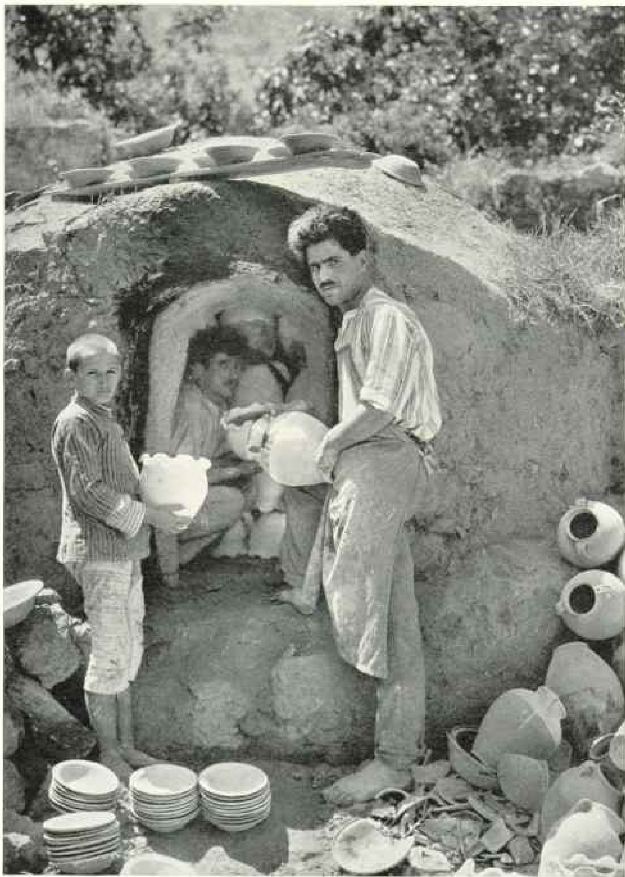
CAREFUL PACKING OF THE KILN INSURES A MAXIMUM LOAD WITHOUT BREAKING
