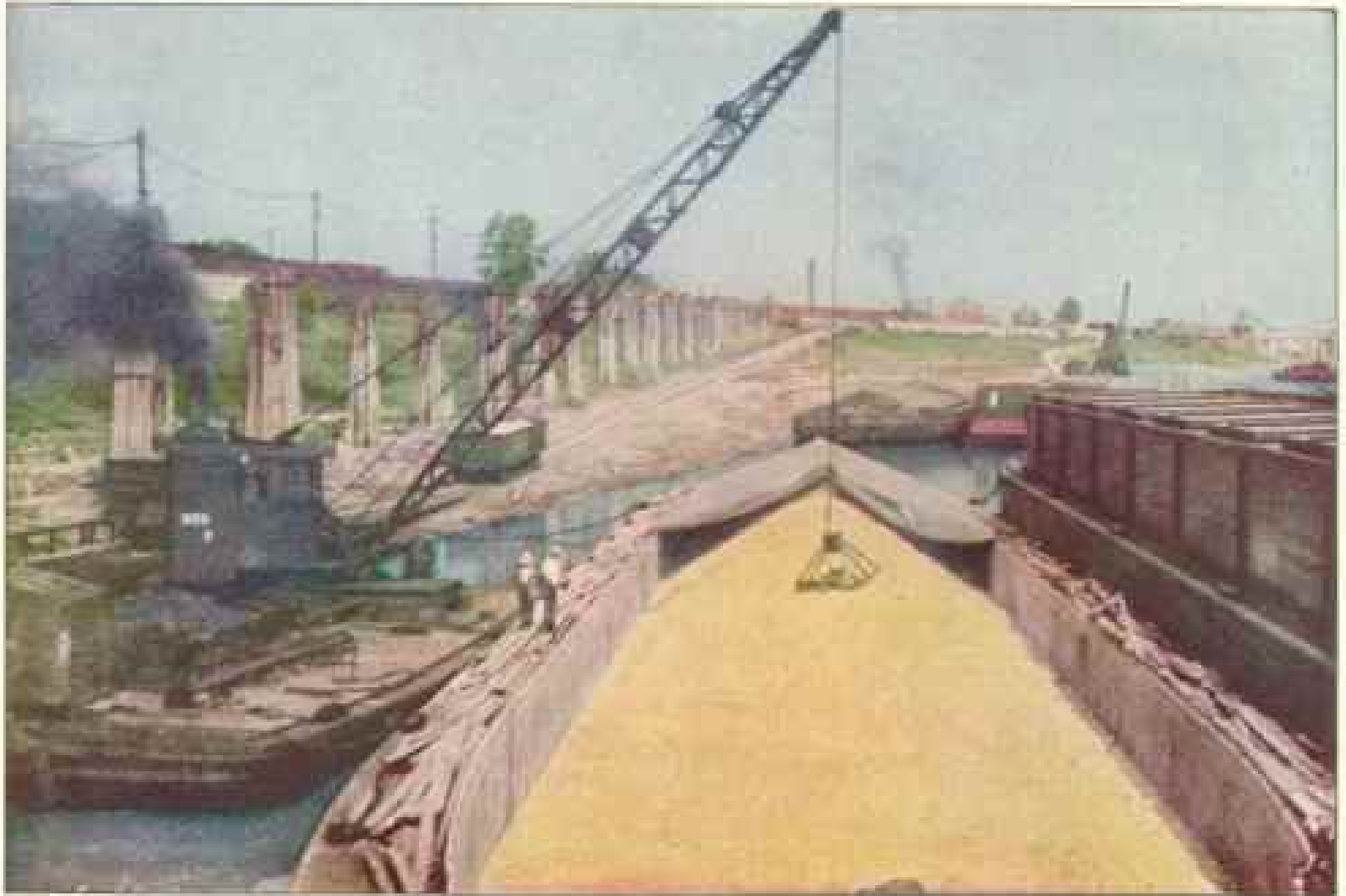
SULPHUR, WATER-BORNE FROM GALVESTON, IS TRANSFERRED TO RAIL AT CAIRO
