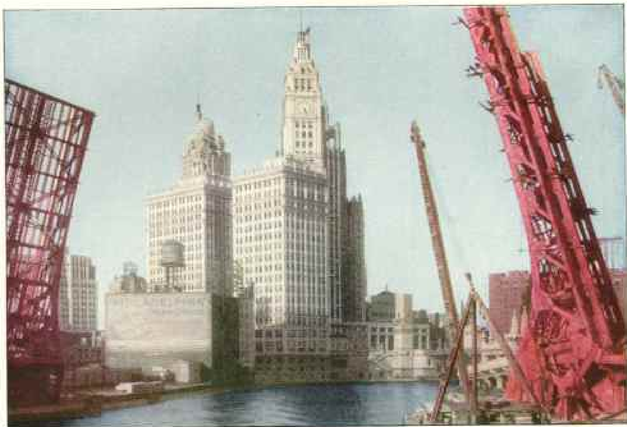
WABASH AVENUE BRIDGE FRAMES A TRIO OF SKYSCRAPERS
