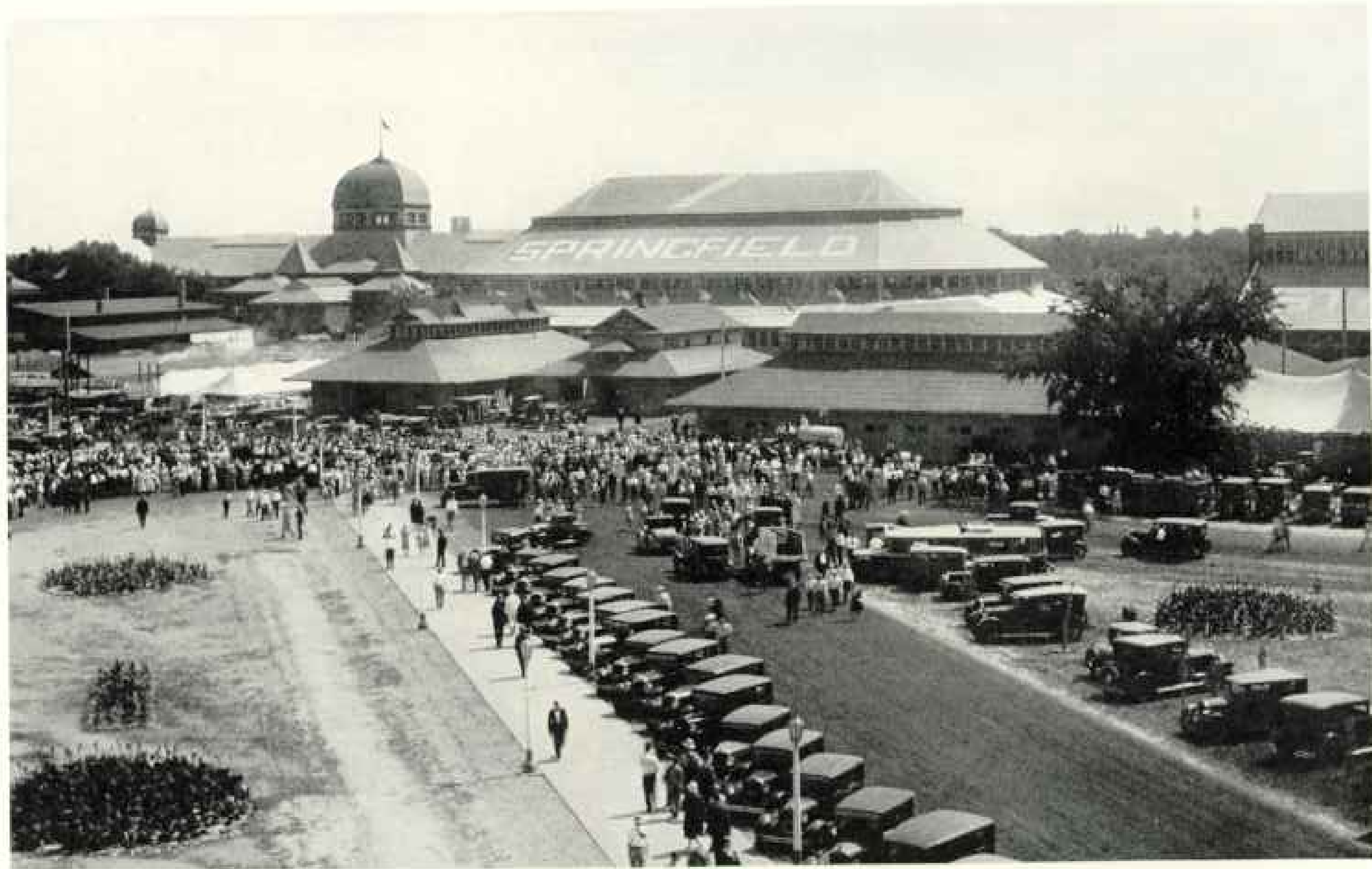
A GROUP OF BUILDINGS OF THE ILLINOIS STATE FAIR AT SPRINGFIELD (SEE, ALSO, COLOR PLATE III)
