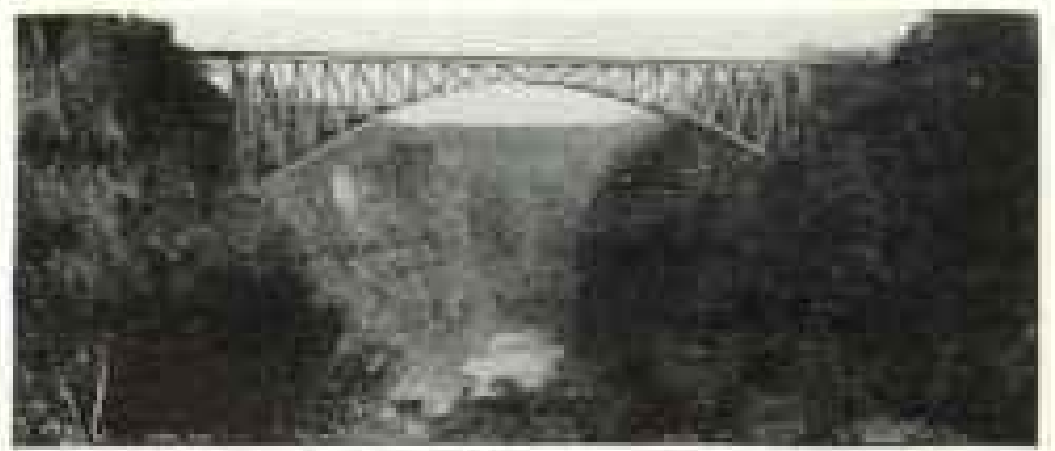
STEEL ARCH BRIDGE, VICTORIA FALLS, AFRICA.
