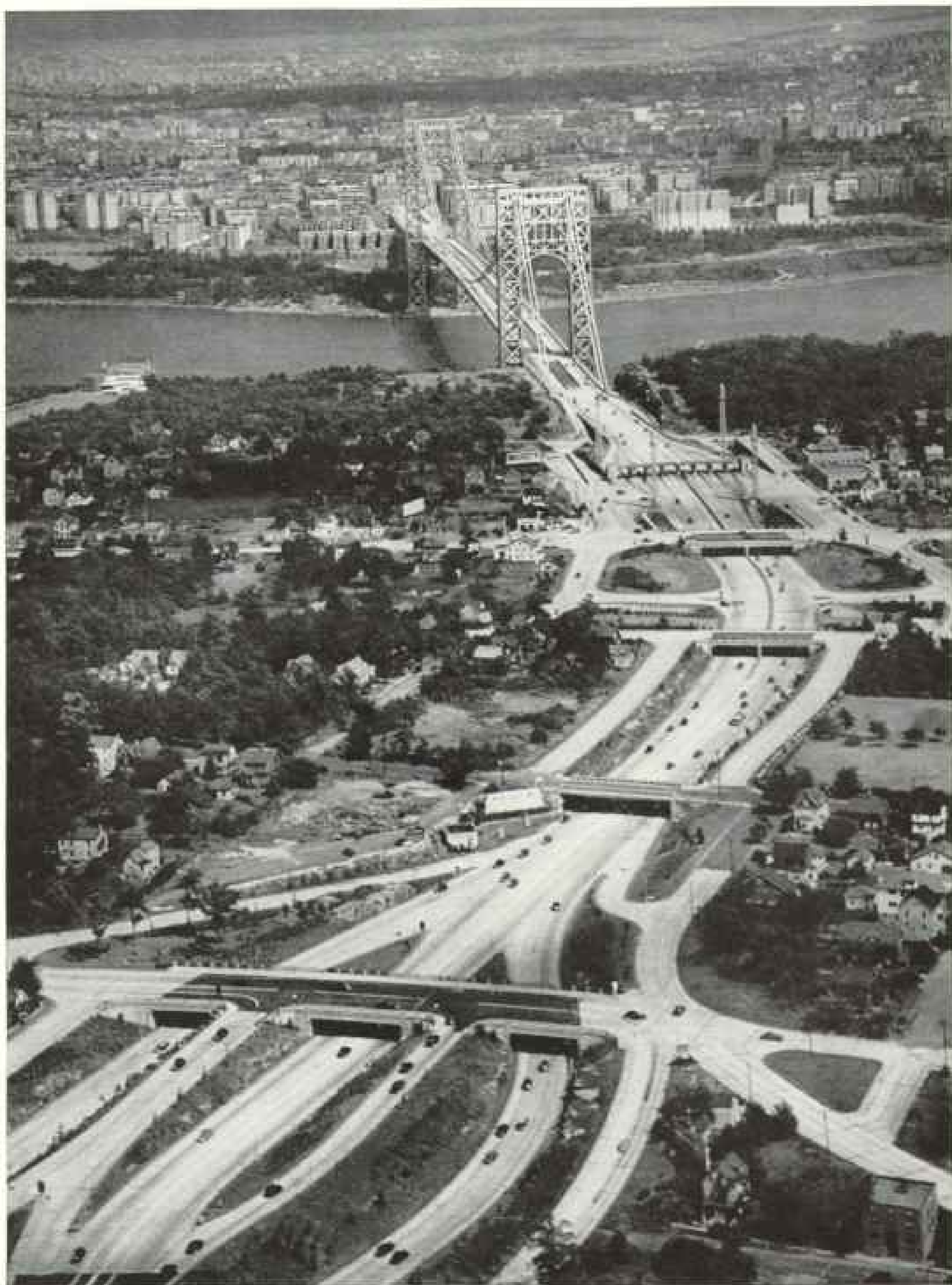
Staff Photographer J. Harlow Roberts from Goodyear Aerially Photographs
